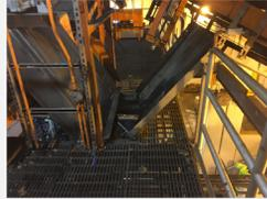
In the E. Rodney French and Cove Rd pump stations, there is no guardrail or sections of the guard have been removed, exposing an employee to a potential fall.
