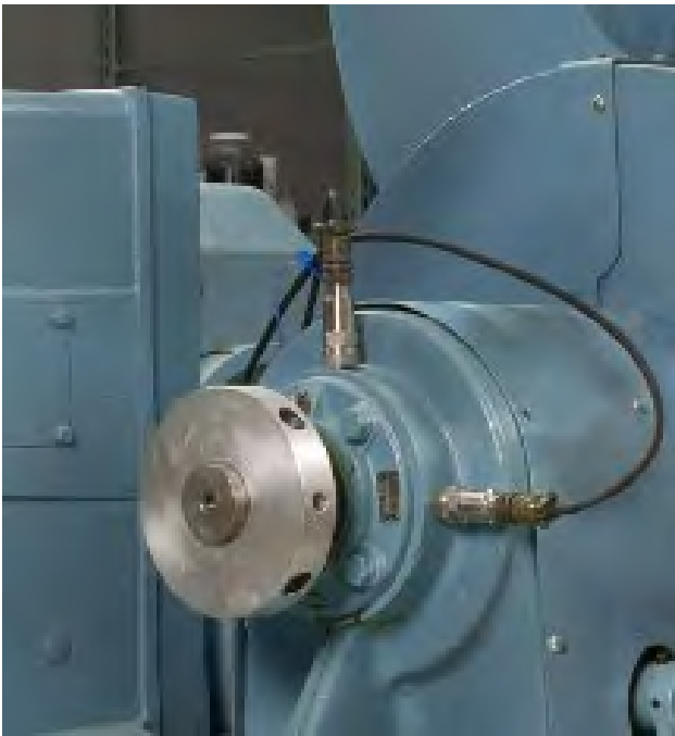
Proper Accelerometer Installation for Predictive Maintenance Analysis
