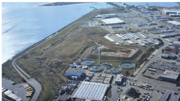
The O&M partnership between the LWSC and Veolia dates back to the startup of their wastewater treatment plant in 1985, and over the past more than three decades this partnership has been recognized with awards, including:
