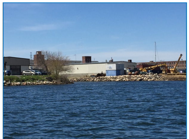
Portions of North Terminal illustrating lack of bulkhead
