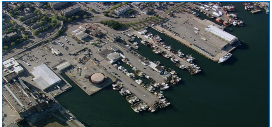
Abundant bulkhead infrastructure at New Bedford's South Terminal. Source: Getty Images
