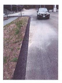
4.) The rip-rap overflow appears to have been set too high. There are no elevations shown on the as-built plan regarding the grading of the raingarden or the overflow.
