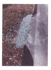
3.) It is unclear whether the access driveway was graded properly. The as-built plan does not show grades along the driveway. Our recollection is the driveway was supposed to be superelevated to direct water towards the raingarden. There is sediment located along the edge of the access driveway opposite the raingarden. If the driveway were superelevated, sediment would not collect on the opposite side of the access driveway.
