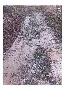
5.) There was evidence of construction vehicles moving within the forebay. This may have been necessary to install the rip-rap overflow. We recommend that the construction vehicle movement in the forebay be limited to prevent compaction of the forebay and allow as much infiltration as possible.
