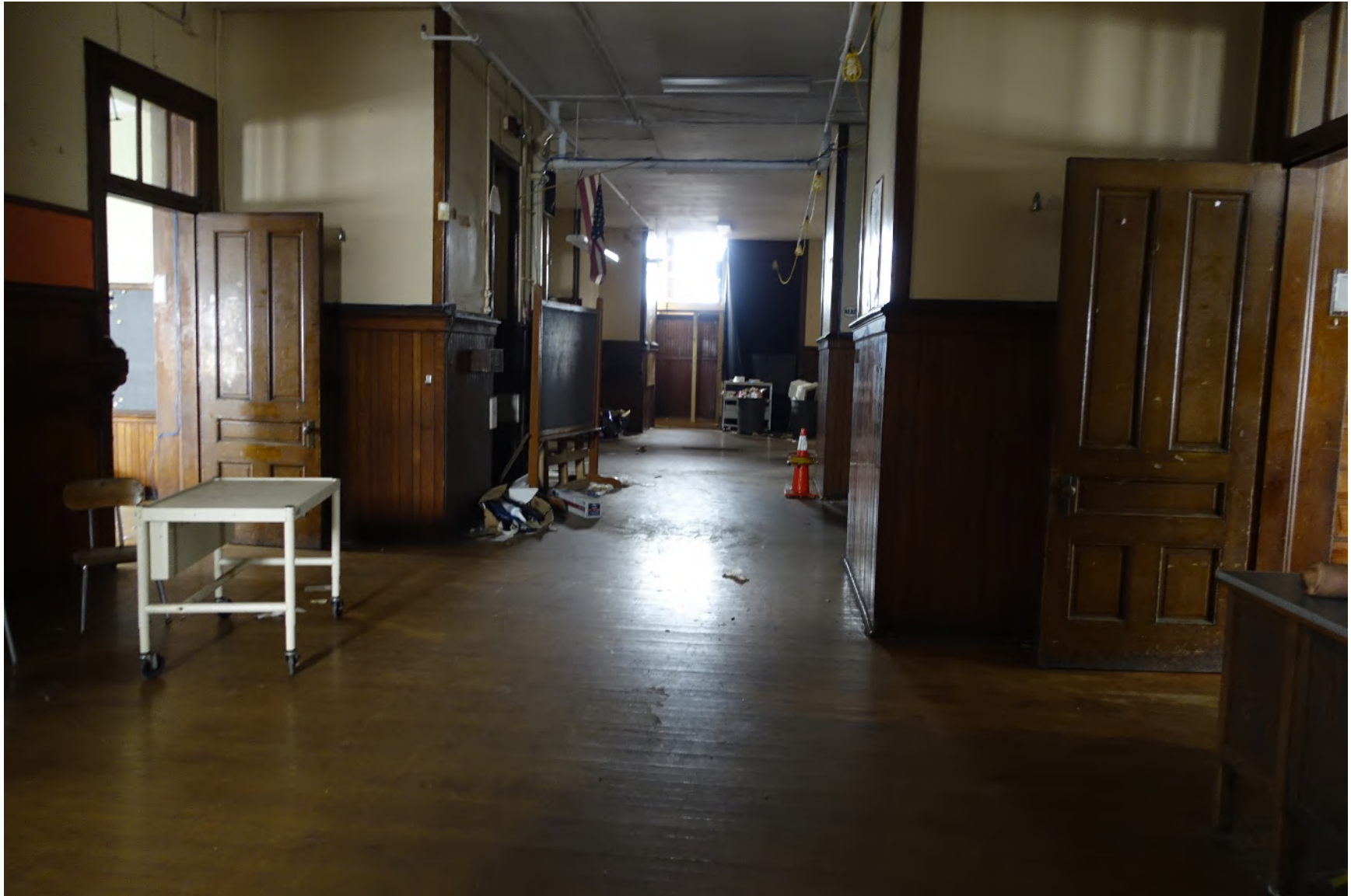
Figure 5-12. First floor interior corridor.
