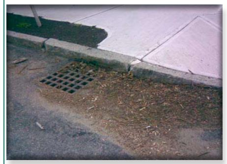
**Description**: Deep sump catch basins, also known as oil and grease or hooded catch basins, are underground retention systems designed to remove trash, debris, and coarse sediment from stormwater runoff, and serve as temporary spill containment devices for floatables such as oils and greases.
