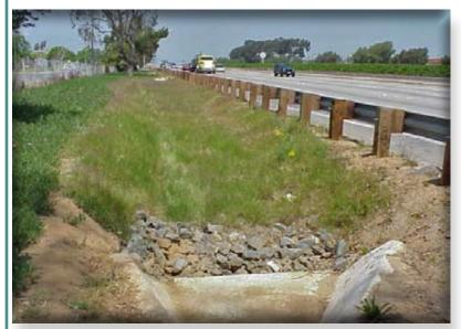
**Description:** Grassed Channels (formerly known as Biofilter swales) are treatment systems with a longer hydraulic residence time than drainage channels. The removal mechanisms are sedimentation and gravity separation, rather than filtration. To receive TSS credit, a sediment forebay or equivalent must be provided for pretreatment. Note that the sediment forebay does not receive a separate TSS removal credit.
