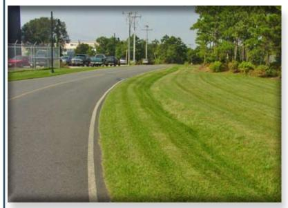
**Description**: Drainage channels are traditional vegetated open channels that are designed to provide for non-erosive conveyance. They receive no infiltration or TSS removal credit (Standards 3 and 4).
