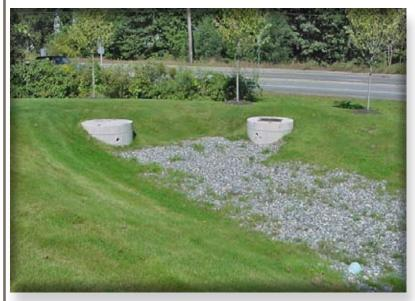
**Description**: Infiltration basins are stormwater runoff impoundments that are constructed over permeable soils. Pretreatment is critical for effective performance of infiltration basins. Runoff from the design storm is stored until it exfiltrates through the soil of the basin floor.
