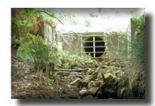
install riprap on the bank opposite the outfall point to protect it from scour.
