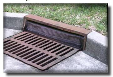
applications. Additionally, larger sized sediment can clog and significantly reduce the effectiveness of some Catch Basin Insert filtering media. Therefore it is important to ensure that flow rates, sediment removal, and the frequency of inspection and maintenance are evaluated.
