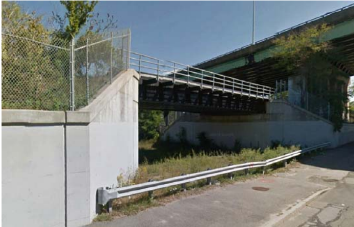
Paso inferior de Purchase Street
