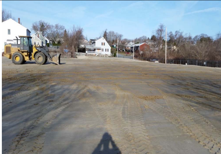
Photo 5: Compacted and graded soil cover/cap at the five contiguous properties.
