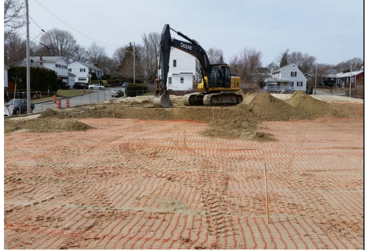
Photo 2: Demarcation layer overlying compacted backfill and geotextile layer.
