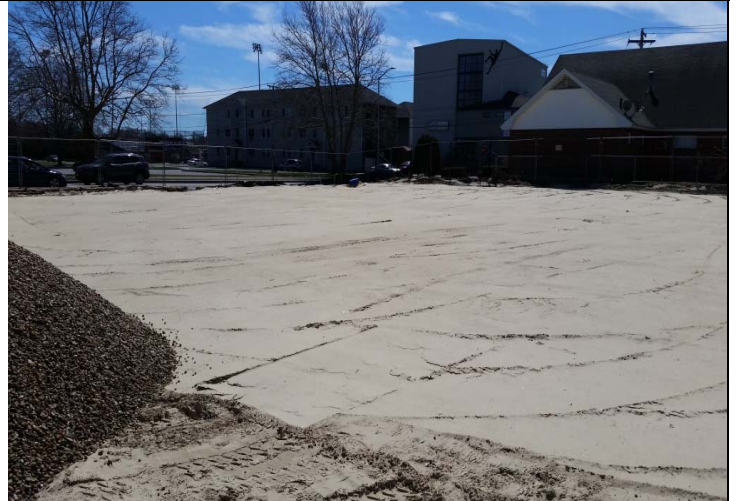
Photo 6: Compacted and graded soil cover/cap at 102 Greenwood Street.
