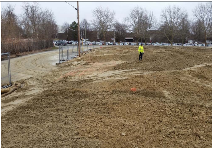
Photo 3: Soil cover prior to compaction.
