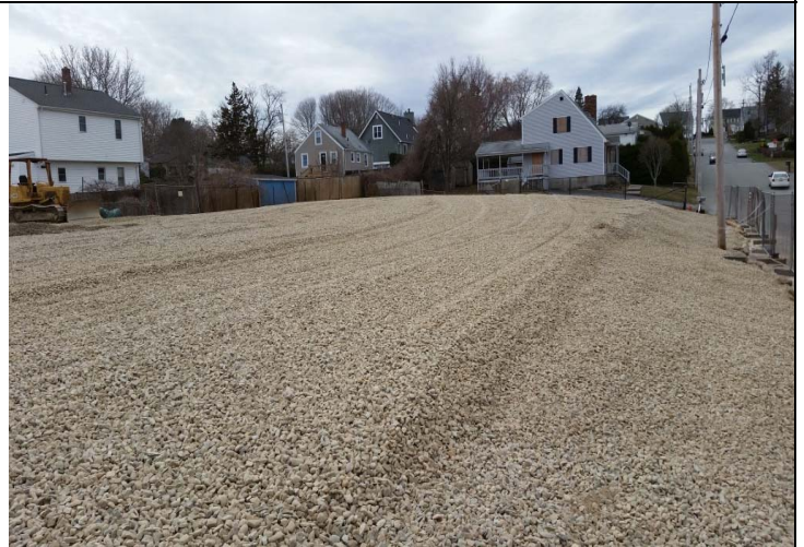
Photo 8: Completed final grade soil cover/cap with crushed stone.
