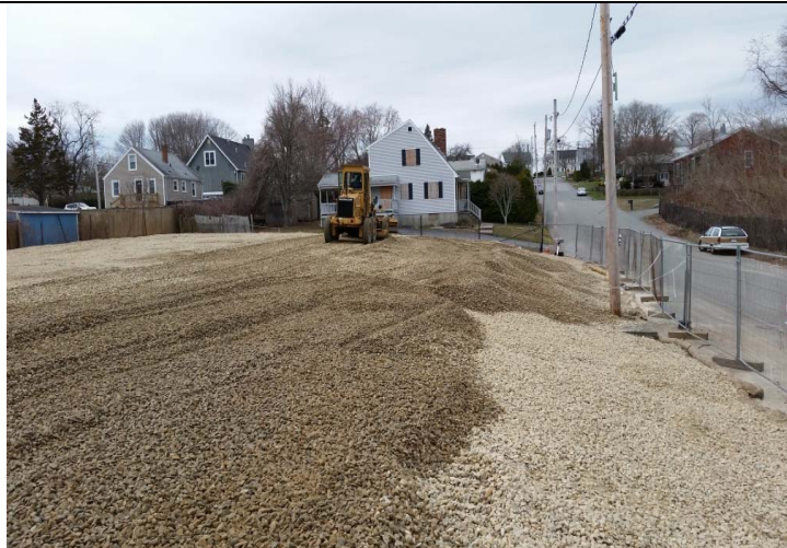
Photo 7: Crushed stone cover installation activities.
