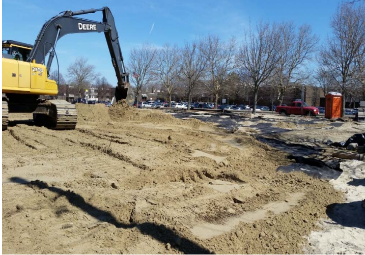
Photo 1: Soil cover/cap installation over black geotextile layer.
