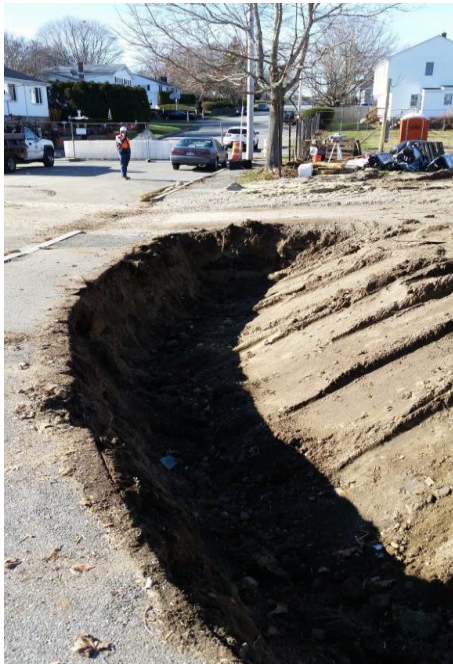
Photo 7: Sloped perimeter excavation in southeast corner of 101 Greenwood Street on December 15, 2014.
