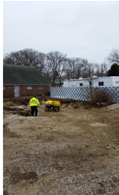
Photo 4: Compacting clean backfill in southwest portion of 102 Greenwood Street on December 8, 2014.
