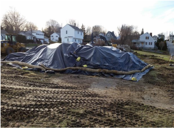
Photo 9: Secured stockpile of non-PCB Remediation Waste soils on December 29, 2014.
