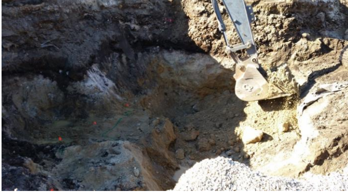
Photo 13: Deeper PCB Remediation Waste excavation at 102 Greenwood Street on January 20, 2015.
