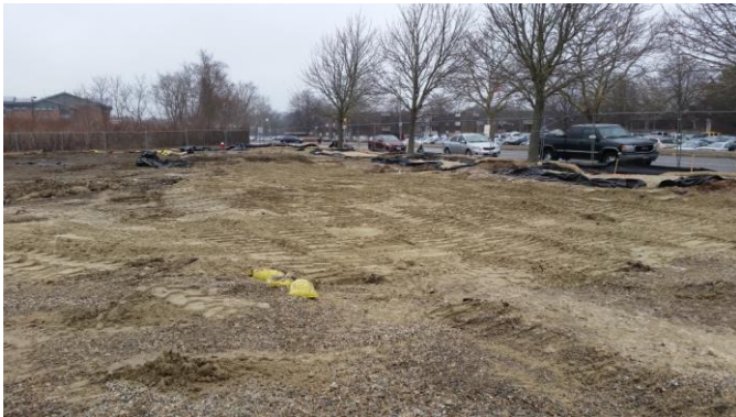
Photo 11: PCB Remediation Waste excavation at 101 Greenwood Street backfilled on January 15, 2015.
