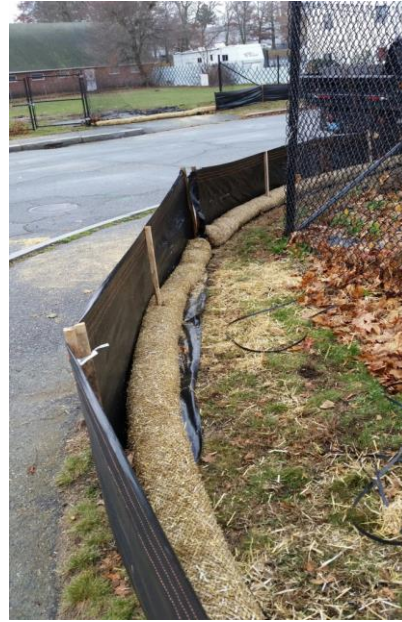
Photo 2: Stormwater controls – silt fence and straw waddle sediment barrier installed around 101 Greenwood Street on November 25, 2014.
