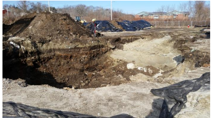
Photo 10: PCB Remediation Waste excavation at 101 Greenwood Street on January 13, 2015.
