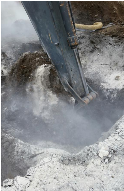
Photo 3: Application of EnviroBlend CS at 101 Greenwood Street on December 2, 2014.
