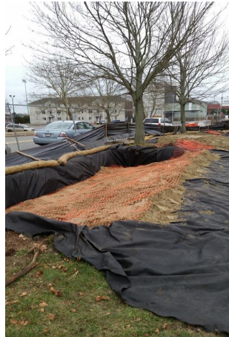
Photo 8: Geotextile fabric, first foot of clean fill, orange warning layer, and tree protection along eastern perimeter of 101 Greenwood Street on December 16, 2014.
