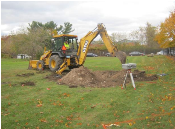
Photo 1: Test pitting around historical boring location SB-101-5A on November 7, 2014.
