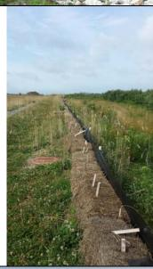
A hay bale check dam was added above the stone apron installed at the end on the RW5 swale. Dewatering of the existing storm drain system to the swale began at 3:00PM
