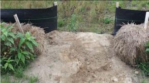
All outlets were inspected to ensure silt fence and hay bales were in place in preparation of the 81-hour shut-down and the pending rain storms. This is the outlet from the area between taxiway A and RW5 runway. The cloudiness and sheen in the ponded water were investigated and appear to be organic in nature.
