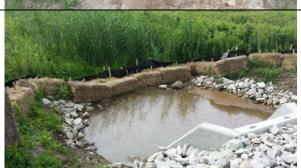
All silt fence on the entire perimeter was inspected. No gaps in fences or hay bale barriers were observed.
