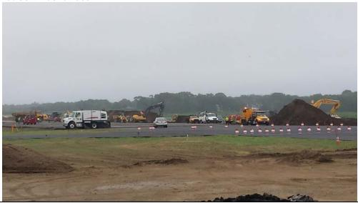
81 hour shut down is well underway by 7:00AM, grinding of pavement has been completed, electrical and storm drain trenches are being dug and loam piles are being shifted out of the area.
