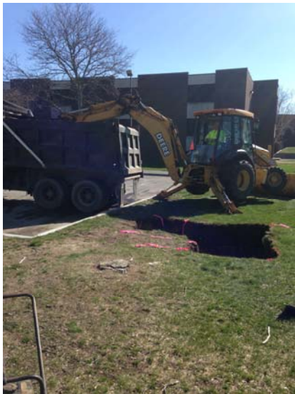
4) View of live-loading of HB-22 soils for offsite disposal facing east (4/24/14).
