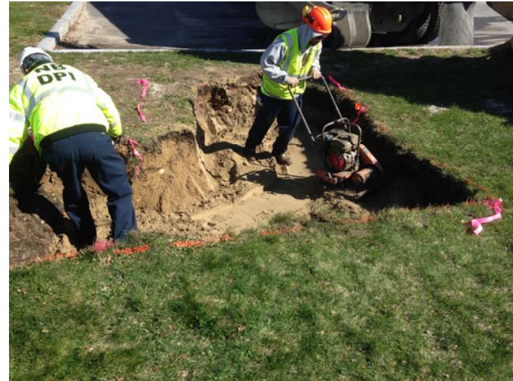
5) View of compaction during backfilling activities (4/24/14).
