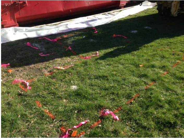
2) View of HB-22 excavation mark-out prior to start of excavation activities (4/24/14).
