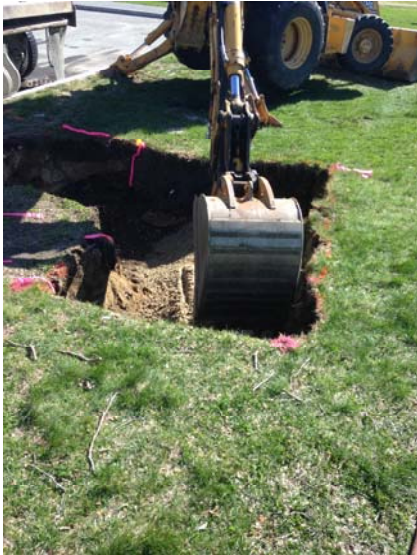
6) Initiation of backfilling of HB-22 excavation (4/24/14).
