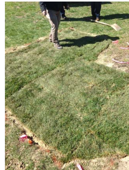
7) View of sod placement at HB-22 (4/24/14).
