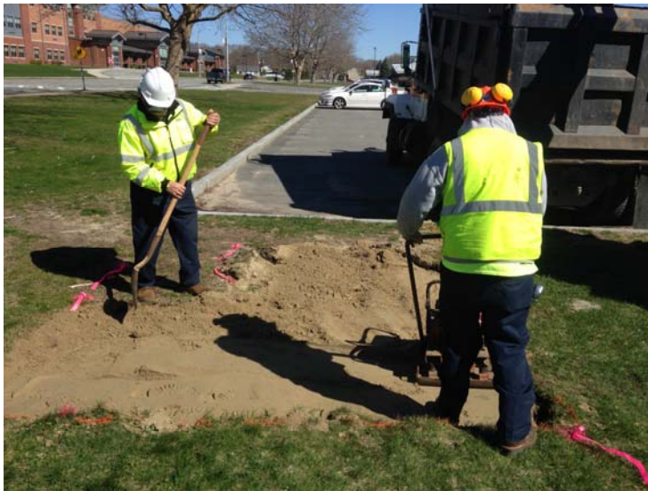
8) View of HB-22 excavation area backfilled to grade facing north(4/24/14).
