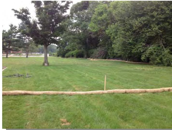
2) Erosion controls viewed to the west (7/9/13).
