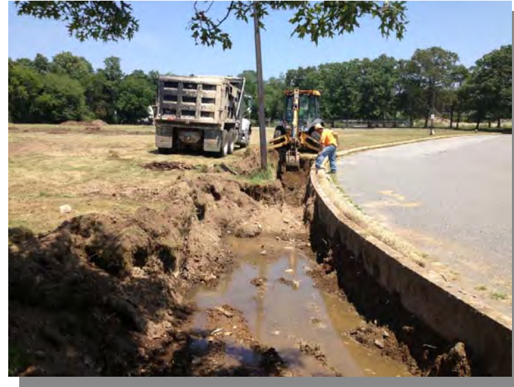
9) Excavation along southern portion of EP HS-8 viewed to the east (7/17/13).
