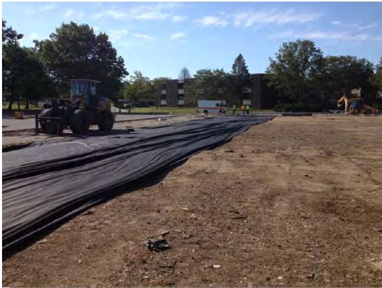
27) Placement of geotextile fabric viewed to the south (8/16/13).
