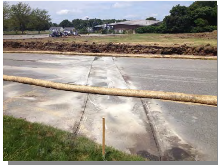
13) Saw cut for conduit trench viewed to the north (7/22/13).
