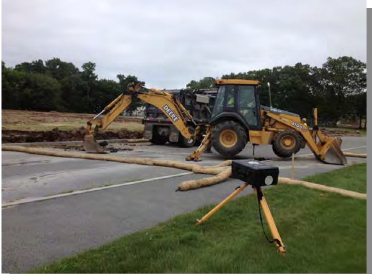
18) Dust monitoring during trench excavation viewed to the northeast (7/25/13).
