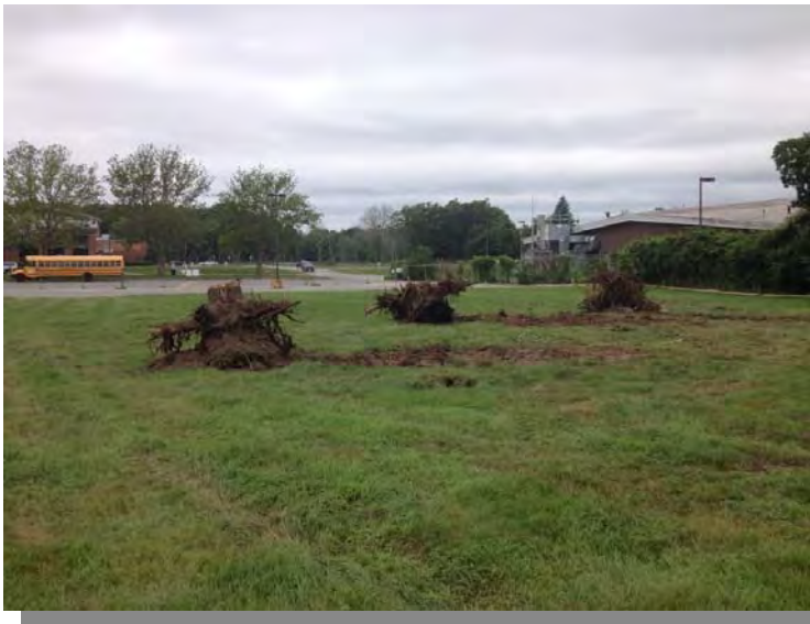
8) Stump removal viewed to the northwest (7/12/13).
