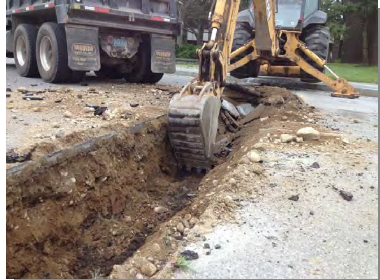
17) Excavation of trench for electrical conduits (7/25/13).
