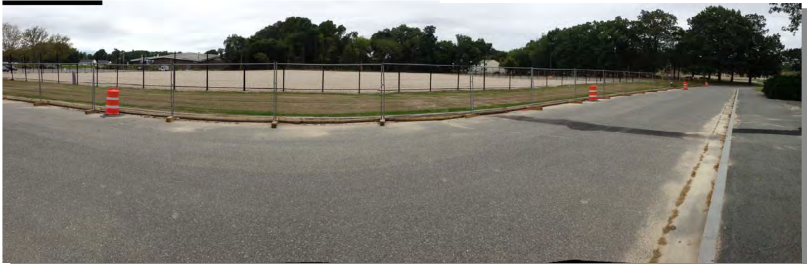
35) View of solar park area following completion of grading activities (9/10/13).
