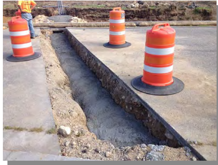
22) Placement of concrete within conduit trench (8/1/13)
