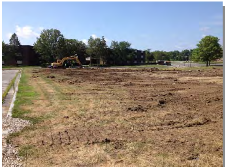
16) Grading of excavated material within solar park footprint (7/24/13).
