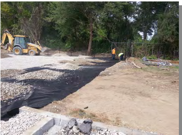
33) Placement of geotextile fabric and stone (8/26/13).
