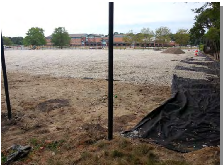
34) Solar park area viewed to the west (8/26/13).
