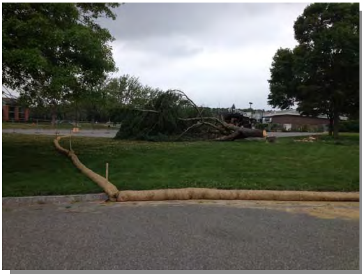
4) Erosion controls and tree removal viewed to the north (7/9/13).
