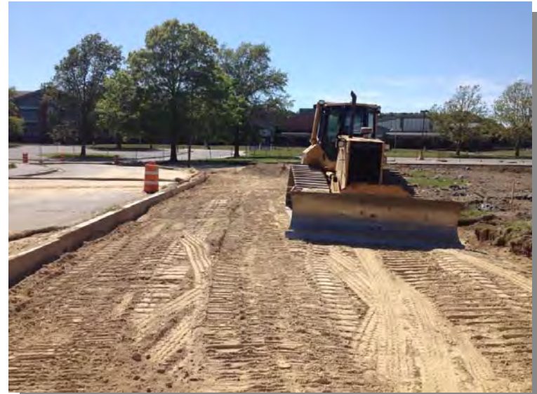
28) Grading activities viewed to the south (8/7/13).
