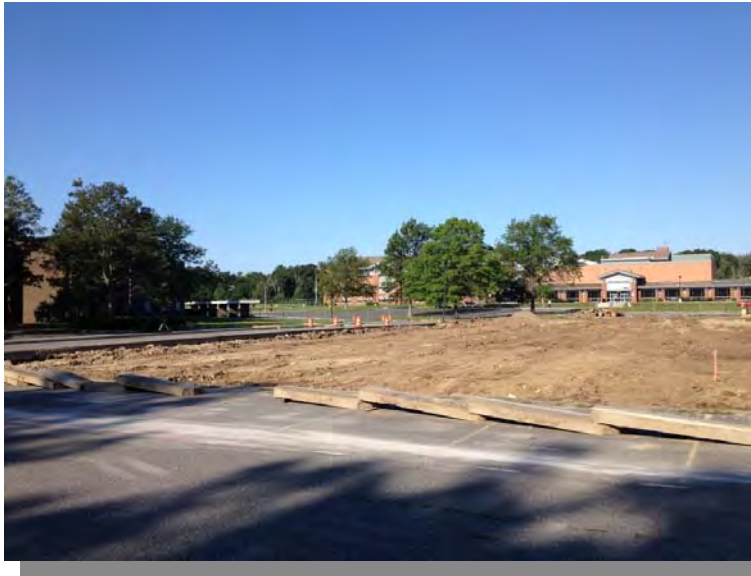
21) Grading of solar park footprint viewed to the west (7/30/13).
