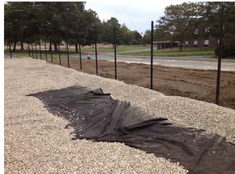
32) Placement of loam viewed to the southeast (8/22/13).
