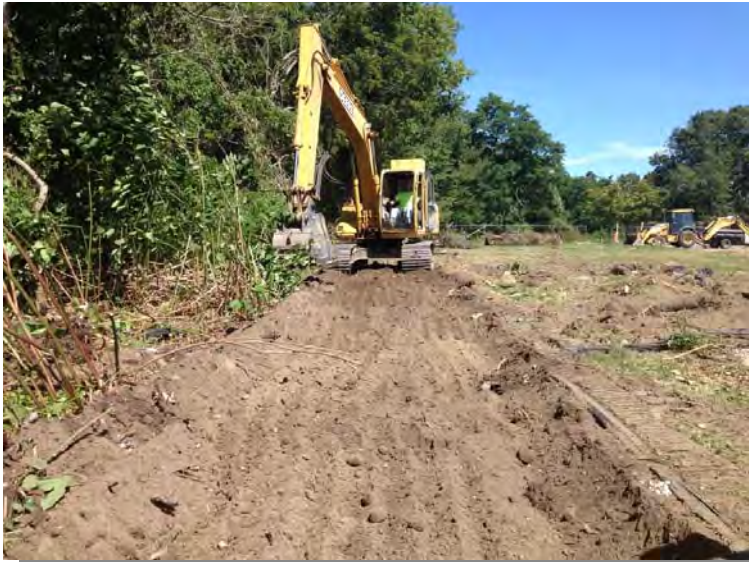
25) Grading along northern property boundary (8/7/13).
