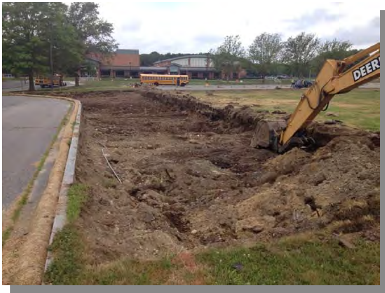
14) Excavation along southern portion of EP HS-8 viewed to the west (7/22/13).
