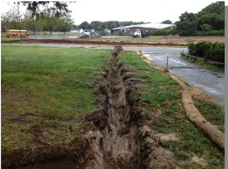
19) Trench excavation for conduits viewed to the north (7/26/13).
