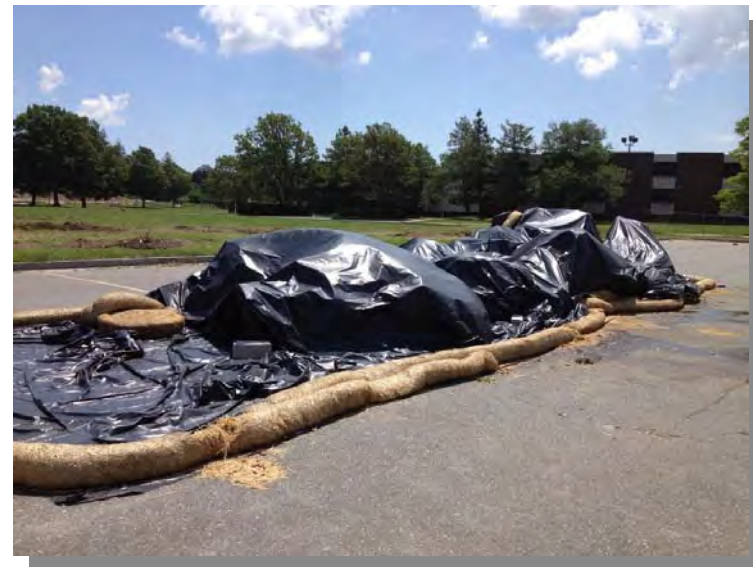
7) Secured stump stockpile viewed to the southeast (7/15/13).
