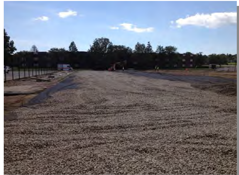
26) Placement of crushed stone viewed to the south (8/16/13).
