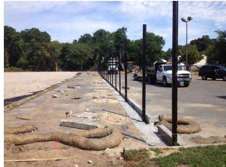
29) Fence installation and placed stone viewed to the north (8/19/13).
