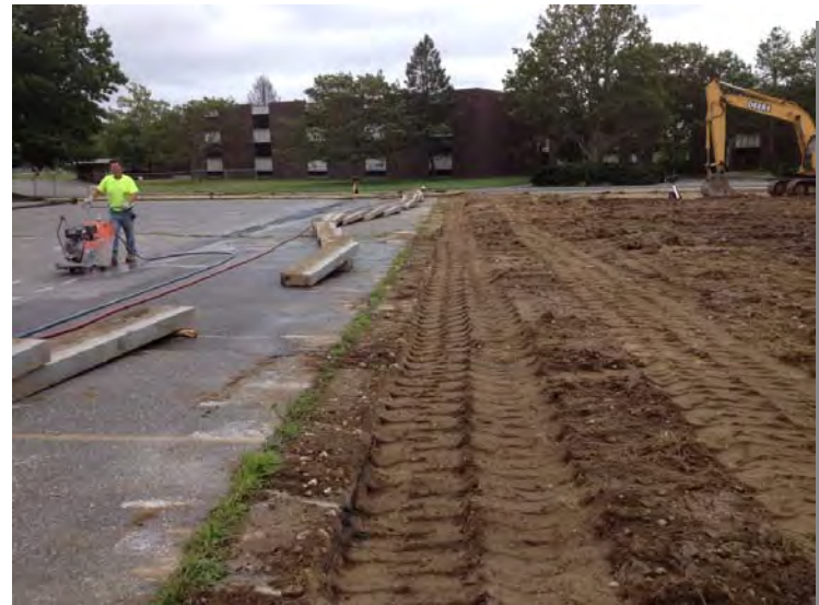
20) Grading and saw cutting for relocation of granite curbing viewed to the south (7/26/13)
