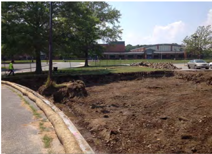
12) Excavation along southern portion of EP HS-8 viewed to the west (7/18/13).
