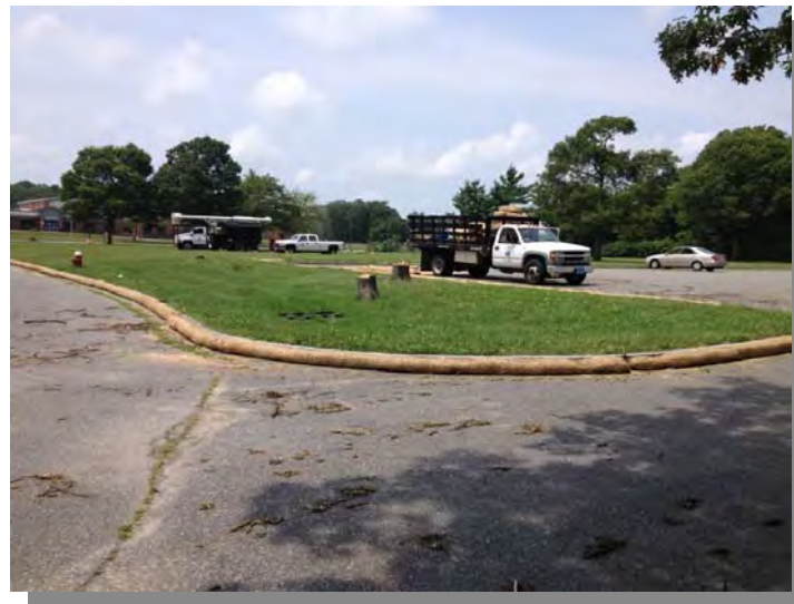
3) Tree clearing and erosion controls viewed to the northwest (7/10/13).
