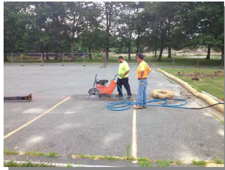
11) Saw cutting northeastern parking lot viewed to the east (7/22/13).
