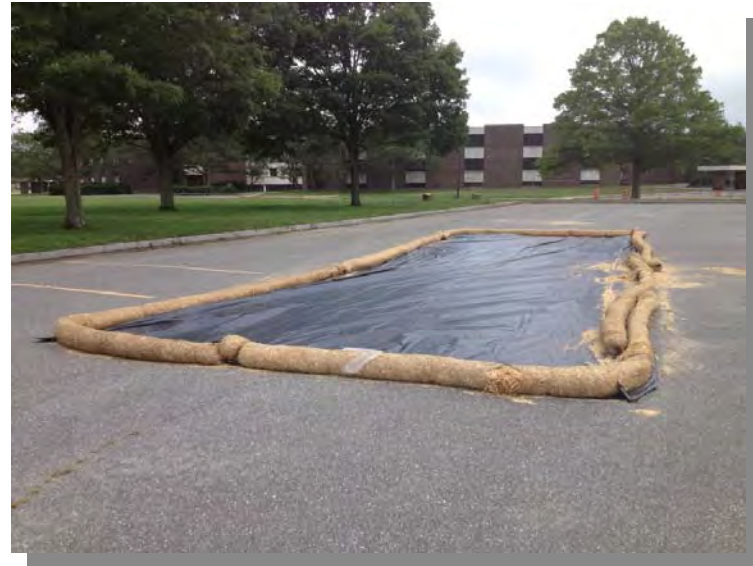
5) Stockpile area viewed to the south (7/10/13).
