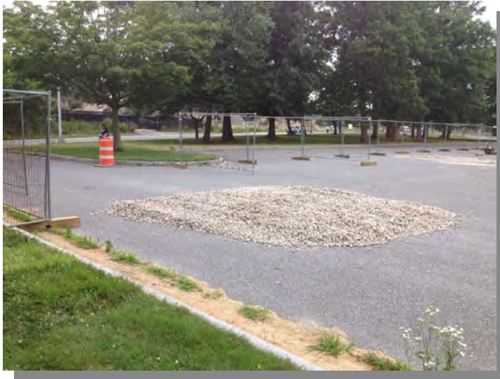
1) Typical construction entrance (7/9/13).
