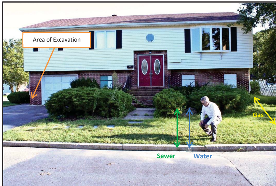
Photo 3 – Subsurface utility locations (102 Greenwood Street)
