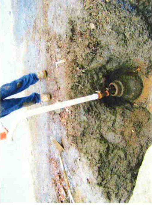
34) DPI flushing air out of blowback valve of water main (11/23/10).
