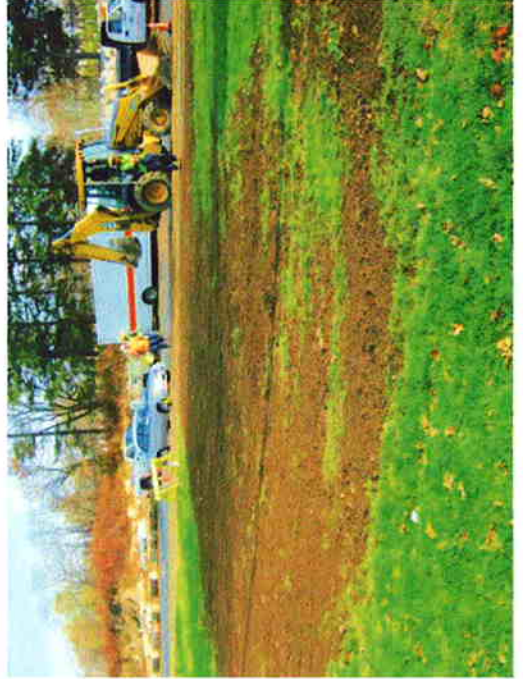
29) Backfilled excavation between Liberty Street and NBHS prepared for loam (11/23/10).
