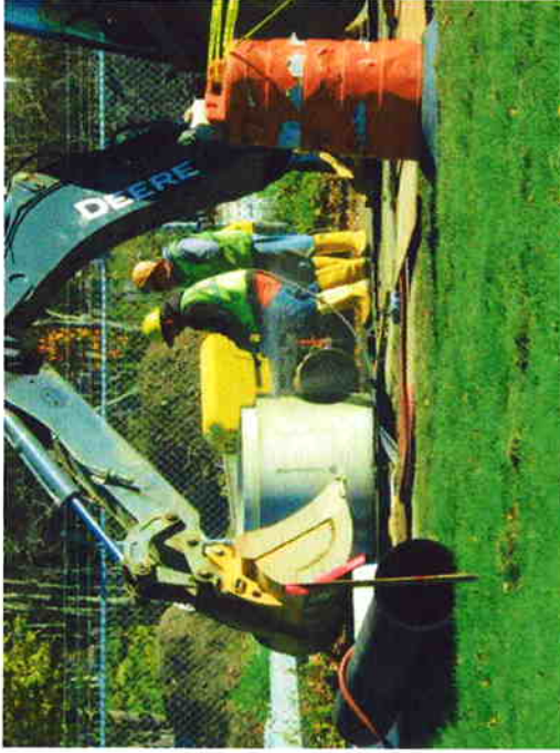
13) Sawing hole in manhole casing to fit drainage pipe (11/12/10).
