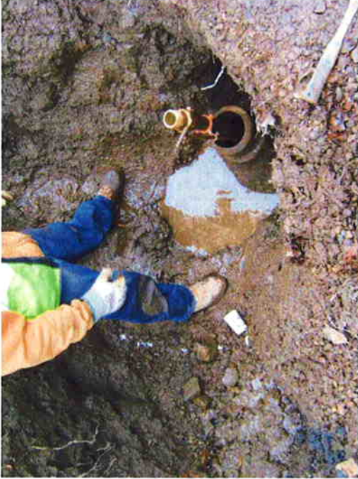
33) Excavation for water main leak (11/23/10).
