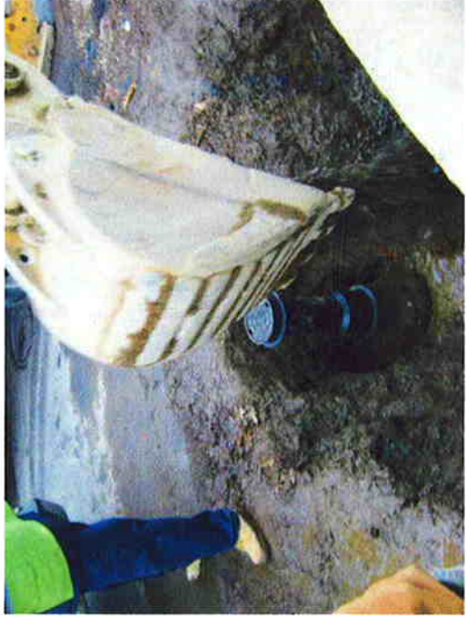
35) DPI backfilling after fitting blowback valve with new casing and cover (11/23/10).
