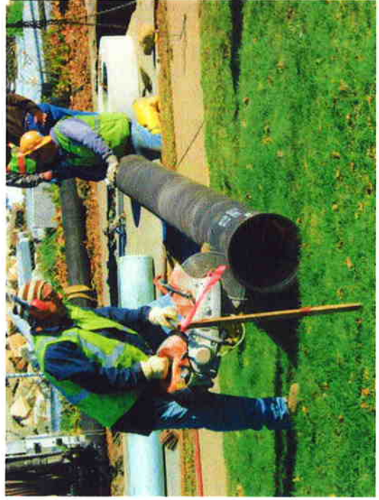
13) Sawing hole in manhole casing to fit drainage pipe (11/12/10).
