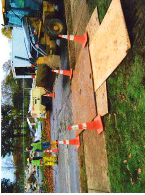
10) Exposed excavation covered at the end of the work day (11/10/10).
