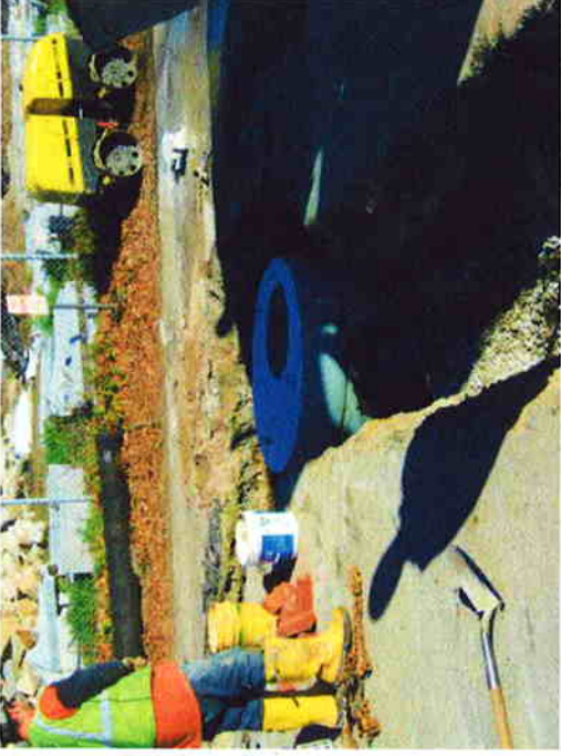
14) Liberty Street manhole in place with drainage pipe attached from west side of street (11/12/10).
