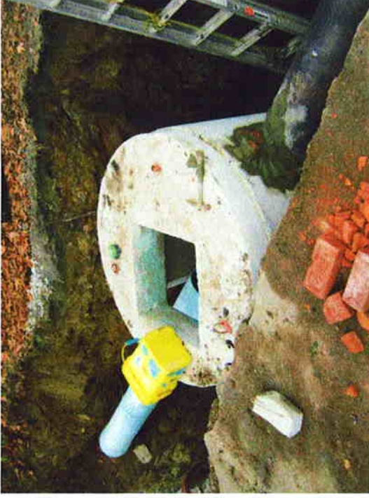
18) Catch basin installation at the eastern edge of Liberty Street (11/15/10).
