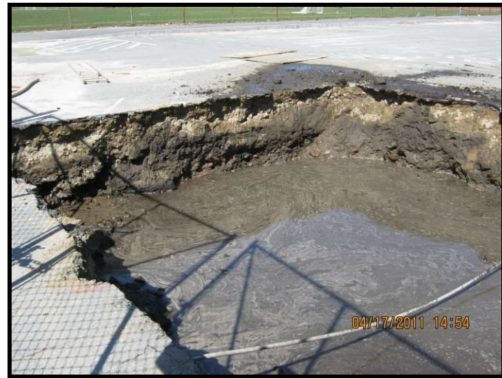
Photo 8 – Groundwater in SB-308 excavation. Dewatered before backfilling (April 17, 2011).
