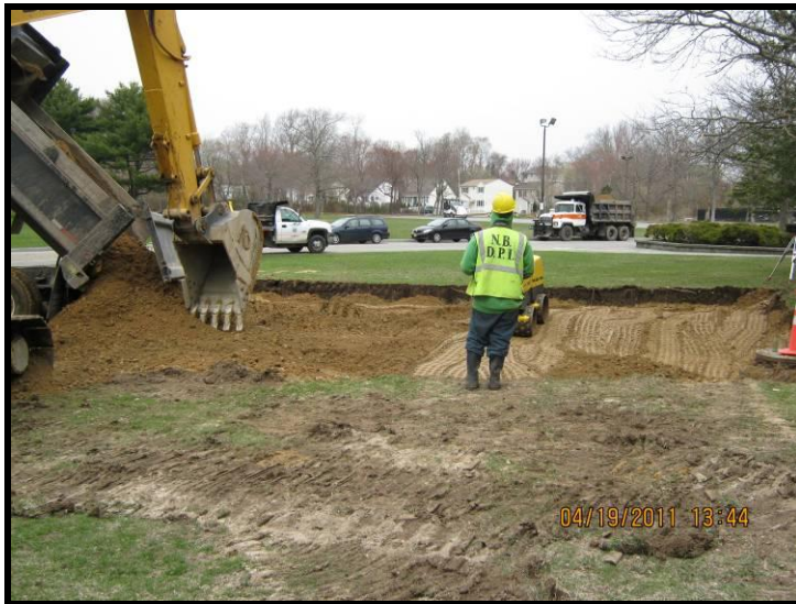
Photo 21 – Backfilling of HH-13 excavation (April 19, 2011).
