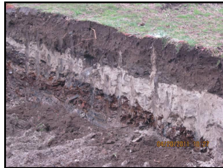
Photo 24 – View of HD-19 excavation (April 20, 2011).
