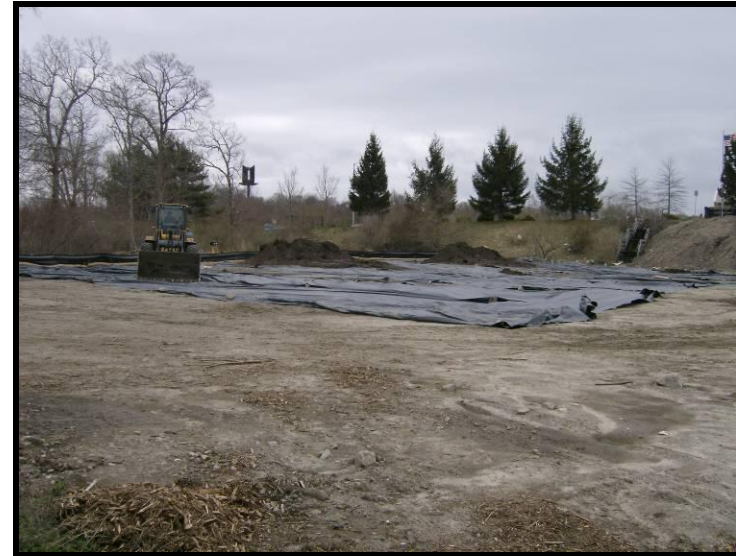
Photo 30 – Polyethylene sheeting for base of stockpiles.
