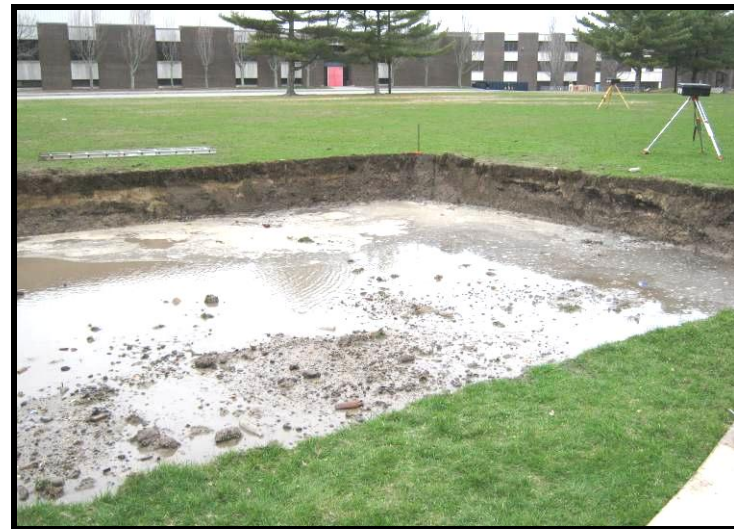
Photo 4 – Excavation SS-36 completed to 3-feet below ground surface (April 16, 2011).
