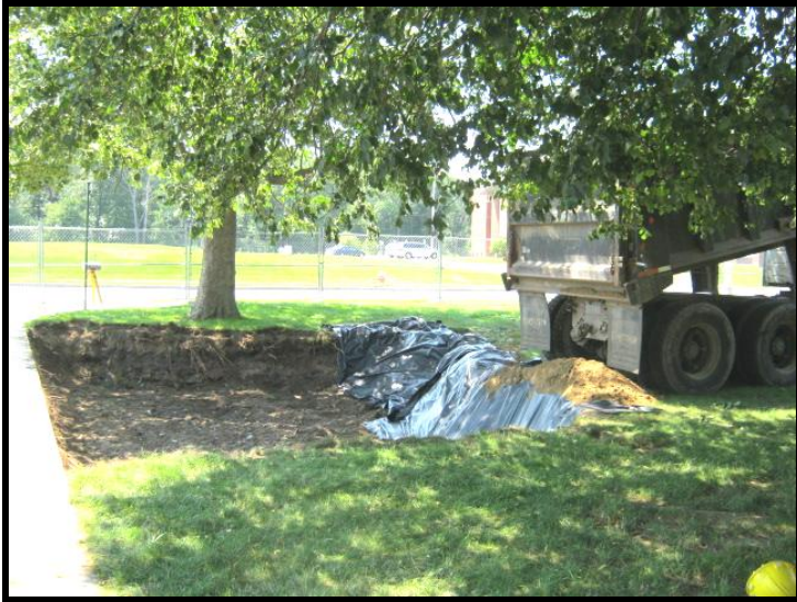
Photo 45 – Portion of HB-23 complete with polyethylene boundary pending further excavation.
