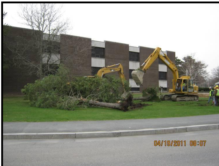
Photo 19 – Removing at HH-13 excavation area (April 19, 2011).
