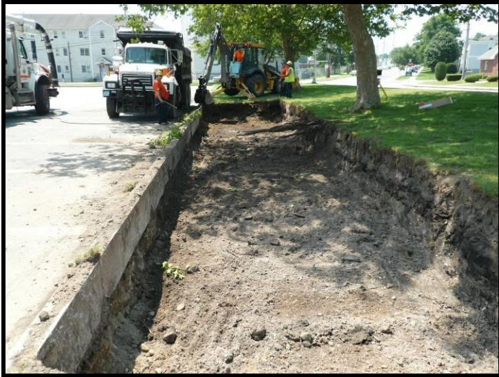
Photo 41 – HB-40 excavation (July 5, 2011).
