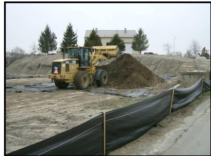
Photo 32– Reworking stockpiles to ensure efficient use of stockpile area.
