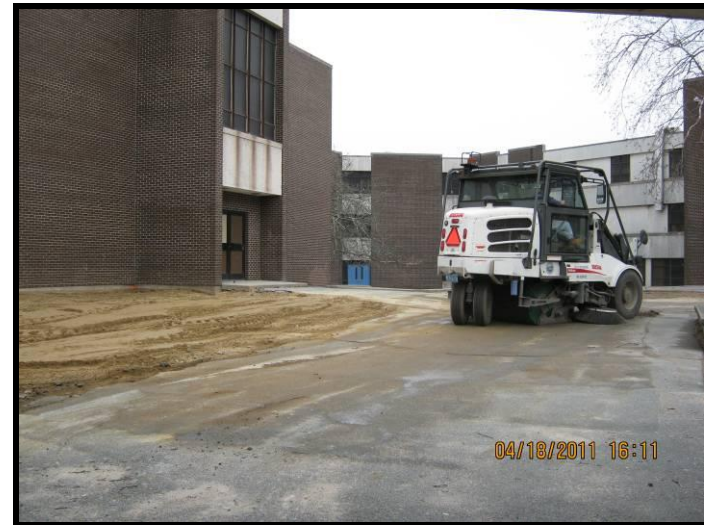
Photo 18 – Street sweeping sidewalk around HF-14 excavation (April 18, 2011).
