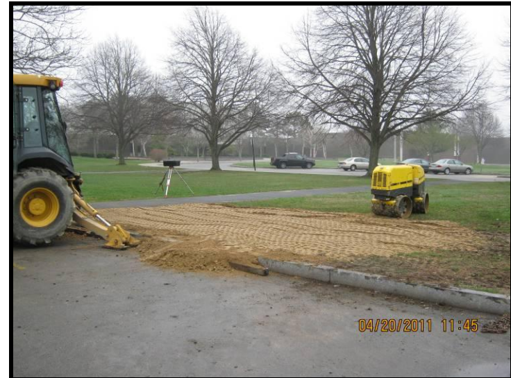
Photo 26 – Completed HC-22 excavation (April 20, 2011).
