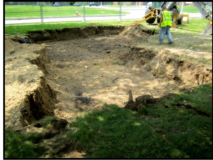
Photo 46 – Portion of HB-23 excavation (July 12, 2011).
