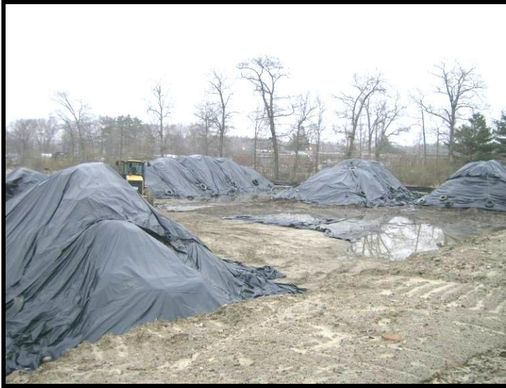
Photo 33- Stockpiles securely covered.
