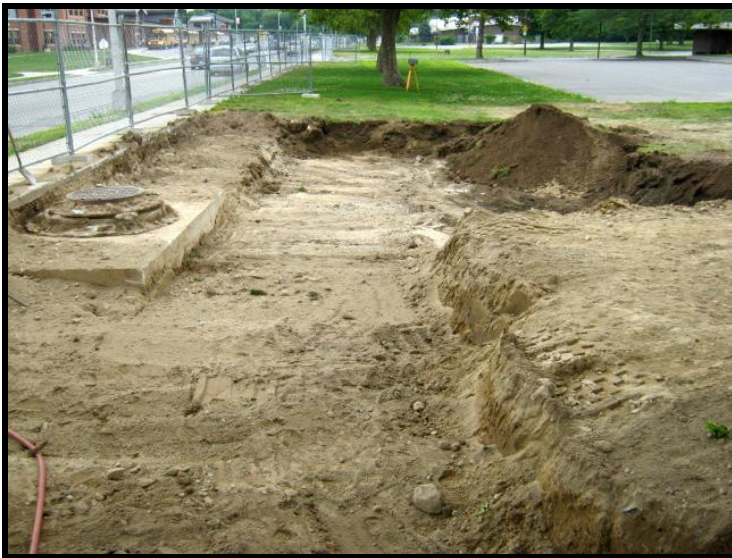
Photo 47 – Remainder of HB-23 excavation (July 13, 2011).
