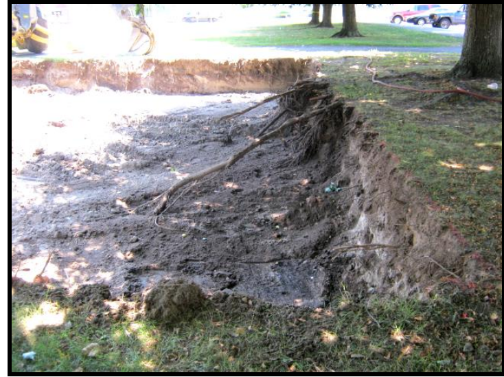
Photo 42 – Tree roots intact inside HF-40 excavation (July 6, 2011).
