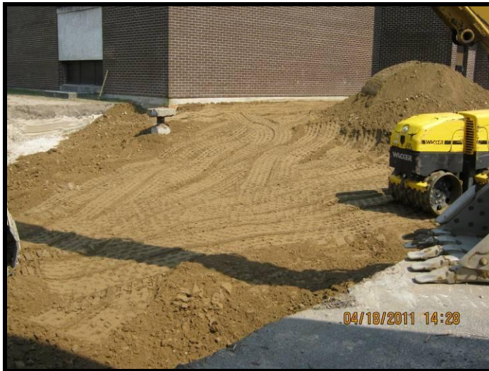
Photo 17 – Compaction between lifts during backfilling (April 18, 2011).
