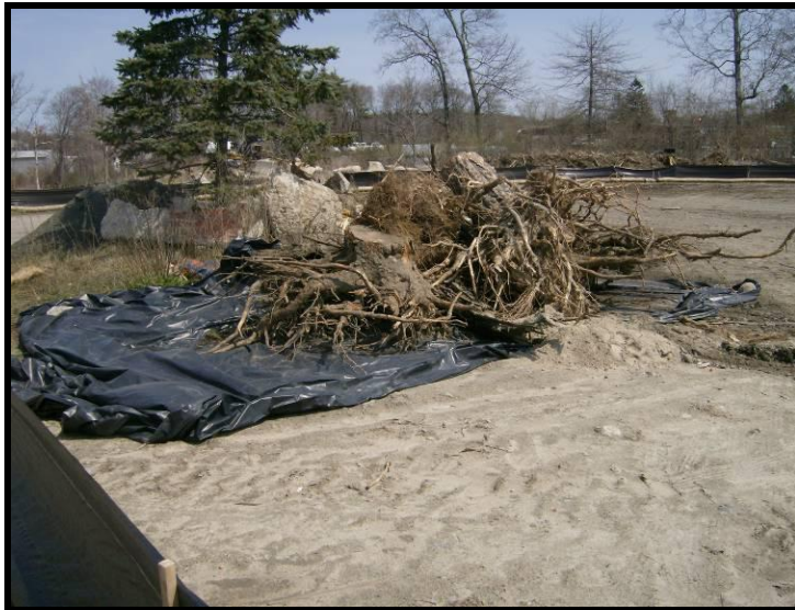
Photo 31- Segregated tree stumps.
