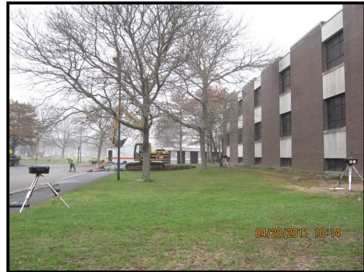
Photo 22 – Active dust monitoring around HD-19 & HD-20 excavations (April 20, 2011).
