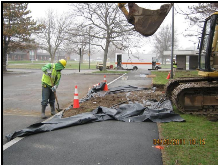
Photo 23 – Polyethylene sheeting collecting soil where trucks are being loaded to keep sidewalk & grass clean (April 20, 2011).
