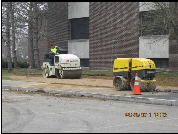
Photo 29 – Rolling backfilled excavations in preparation for loaming (April 20-21, 2011).
