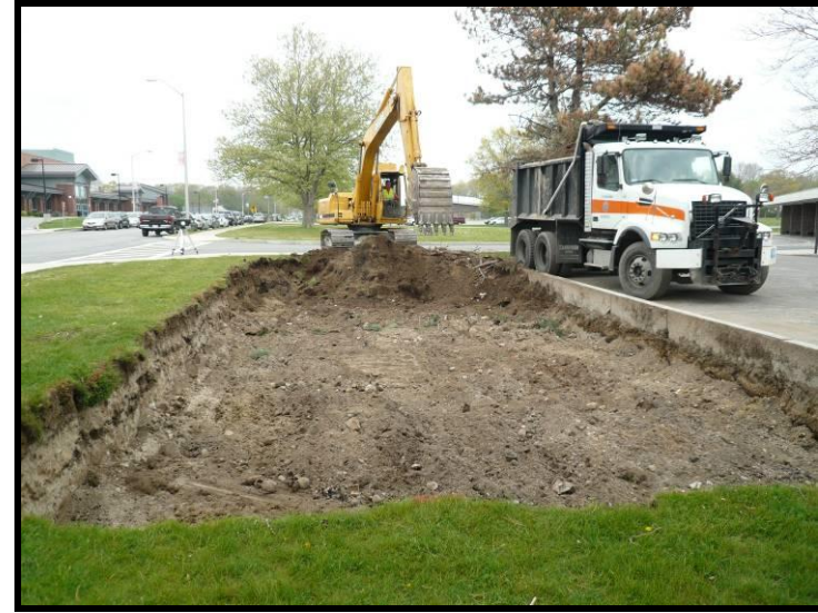
Photo 34 – Excavation activities at HA-19 location (May 14, 2011).
