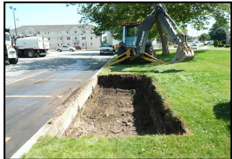
Photo 40 – HB-39 excavation (June 27, 2011).
