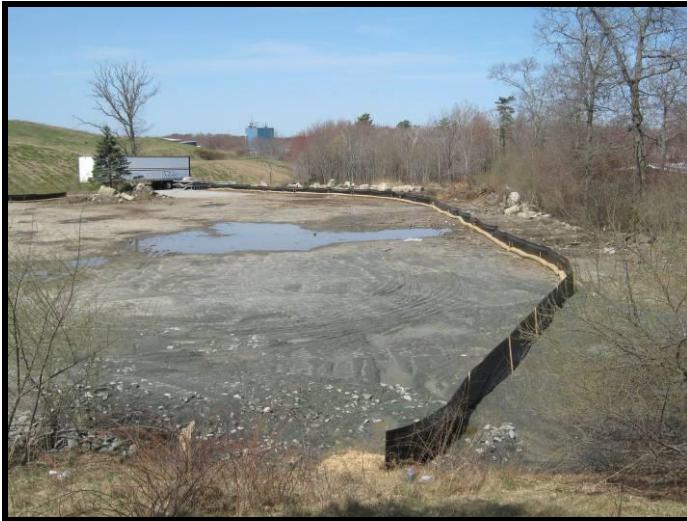
Photo 1 – Preparation of Transfer Station stockpile area in advance of work (April 15, 2011).
