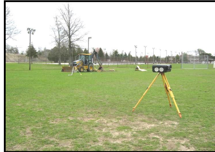
Photo 2 – DustTrak units set up to monitor fugitive dust levels (April 16, 2011).
