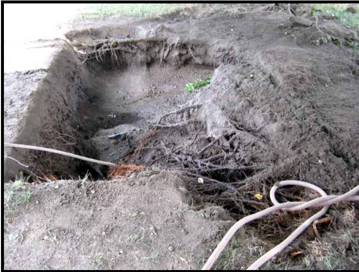
Photo 43 – Air knifing through roots at HF-43 location (July 7, 2011).
