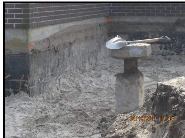
Photo 16 – Sewer cleanout intact in HF-14 (April 18, 2011).
