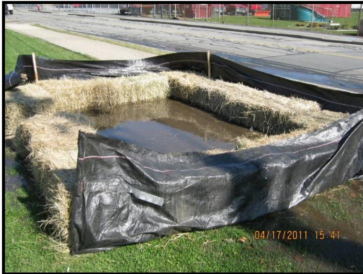
Photo 9 – Dewatering trap consisting of hay bales and silt fence to collect silt from water pumped from SB-308 (April 17, 2011)
