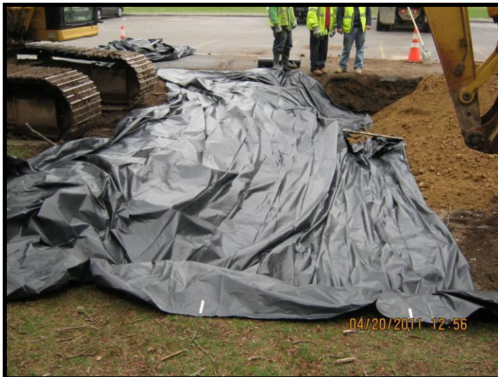
Photo 27 – Polyethylene sheeting over extent of HD-20 excavation toward the south (April 20, 2011).
