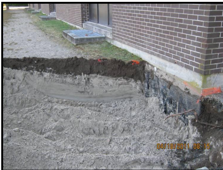
Photo 15 – HF-14 excavation exhibiting topsoil and a tan fine sand (April 18, 2011).
