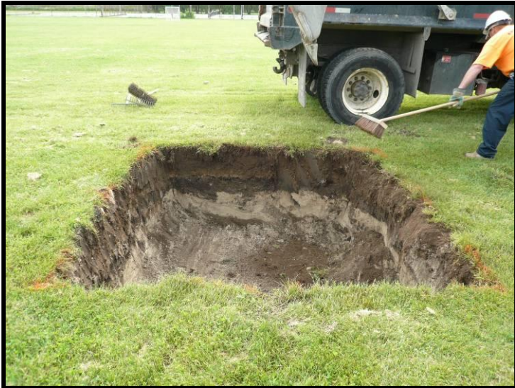
Photo 37 – SS-32 excavation (June 20, 2011).
