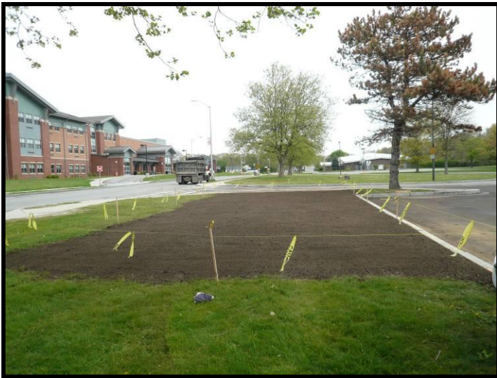
Photo 35 – Completed HA-19 excavation (May 15, 2011).
