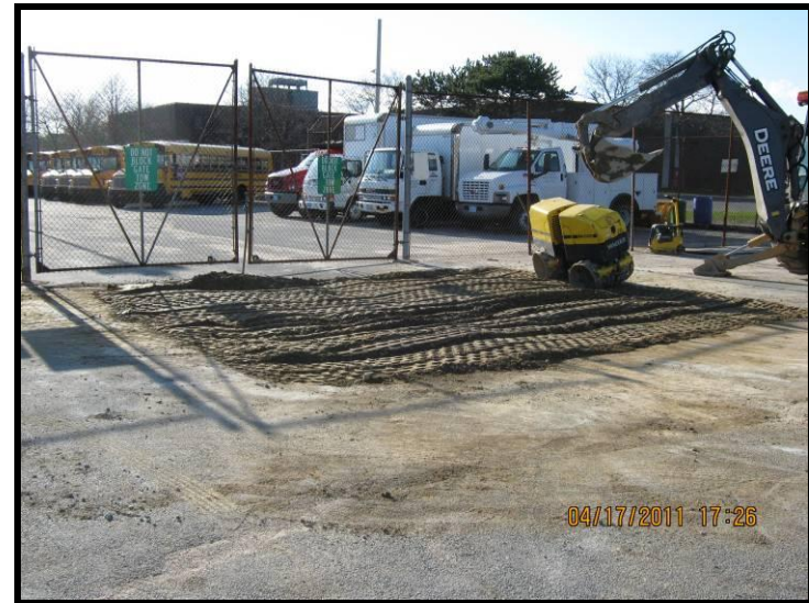
Photo 14 – Completed backfilling of SB-308 (April 17, 2011).
