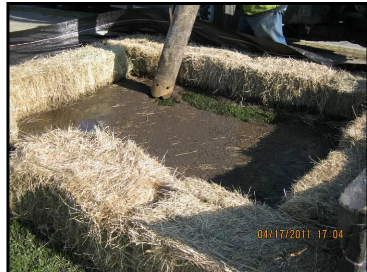
Photo 12 – Vacuum removal of material from trap used for dewatering (April 17, 2011).
