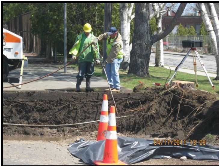
Photo 7 – Using Air Knife to excavate around utilities (April 17, 2011).
