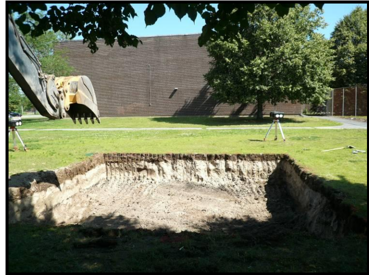
Photo 38 – HJ-42 excavation (June 27, 2011).
