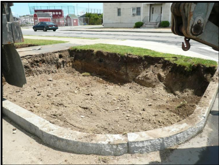
Photo 39 – HE-44 excavation (June 27, 2011).
