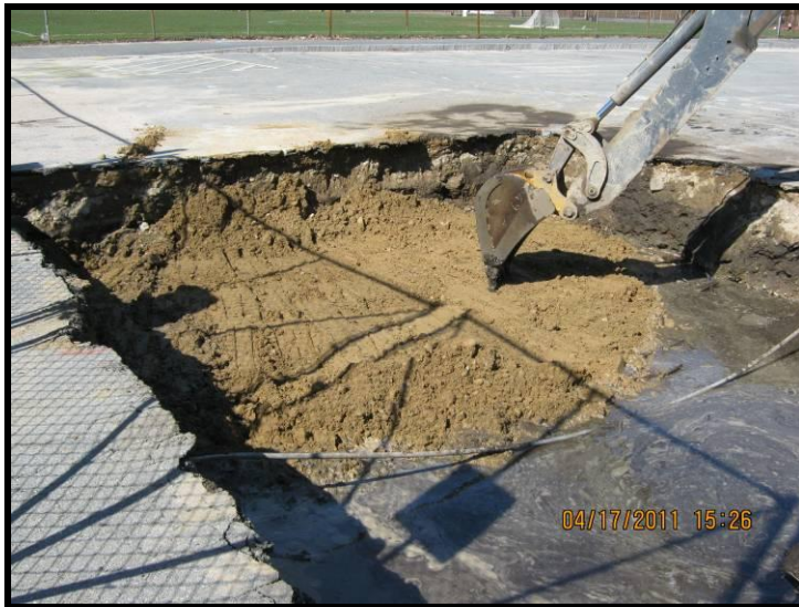
Photo 13 – Backfilling SB-270 in approximately 12-inch lifts (April 17, 2011).
