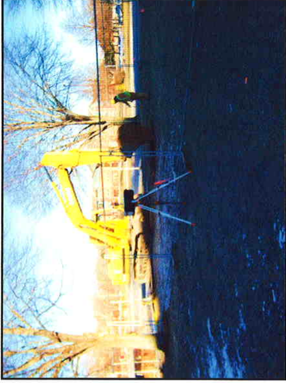
2. Excavation of PCB Remediation Waste soil (February 23, 2011).
