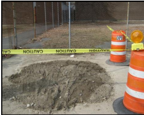
Photo 5: Close up of backfilled excavation area (view from the south).
