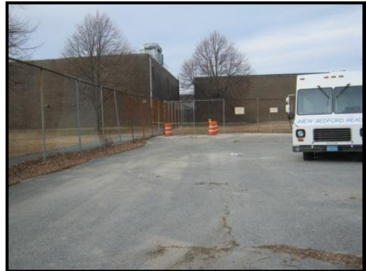
Photo 6: Area of water main repair within the Bus Yard (view from the south).
