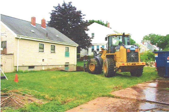
13. Moving decontaminated plates to access 111 Greenwood Street parcel (7/23/10).
