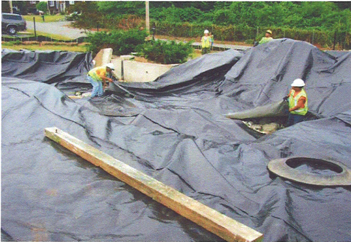
9. Exposed foundation at 118 Ruggles Street covered at end of work day (7/21/10).
