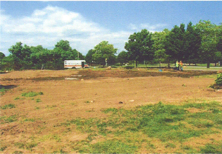
19. Finished grading in area of 98 Ruggles Street & 101 Greenwood Street parcels (8/2/10).
