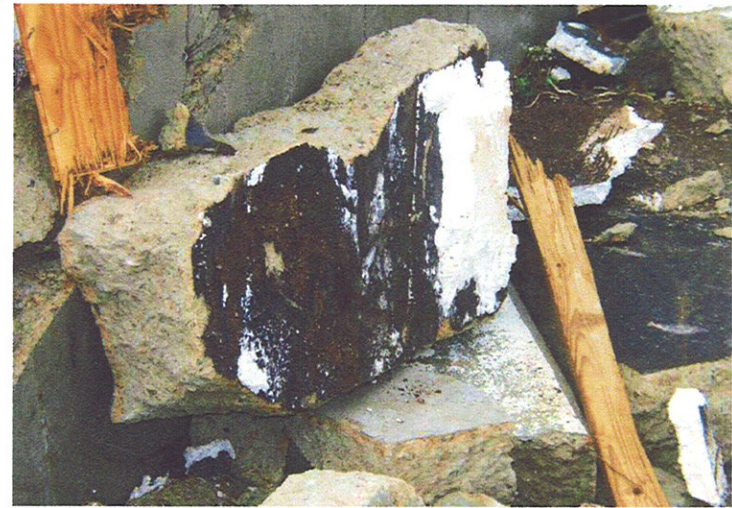
10. Foam insulation adhered to concrete at 118 Ruggles Street (7/21/10).
