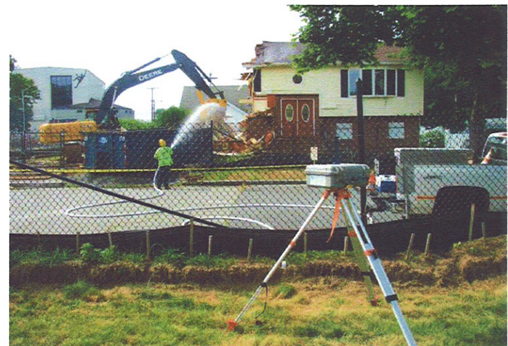
4. DustTrak recording ambient dust levels during demolition activity (7/19/10).
