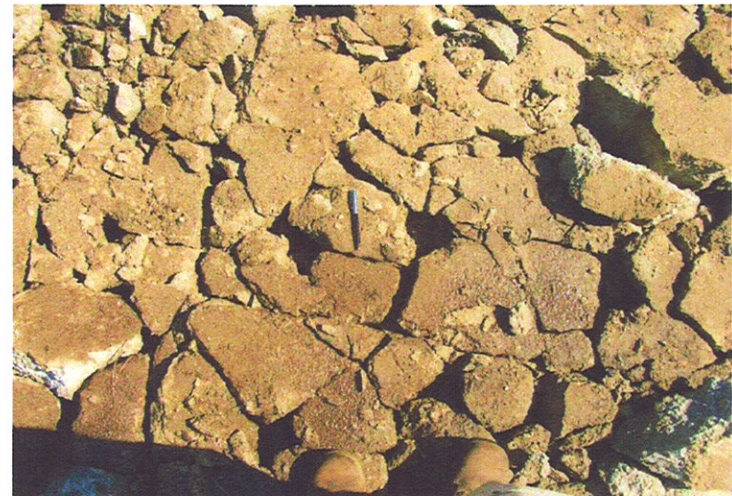
16. Concrete broken to 6-inch minus (7/27/10).
