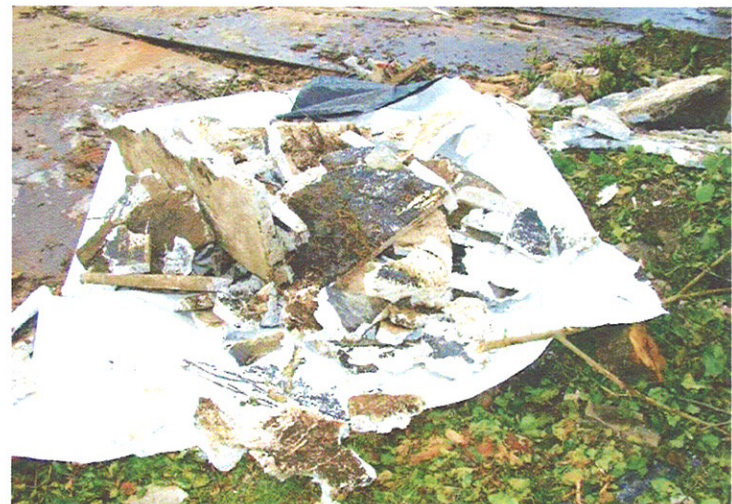
12. Foam insulation from 118 Ruggles Street for offsite disposal (7/22/10).
