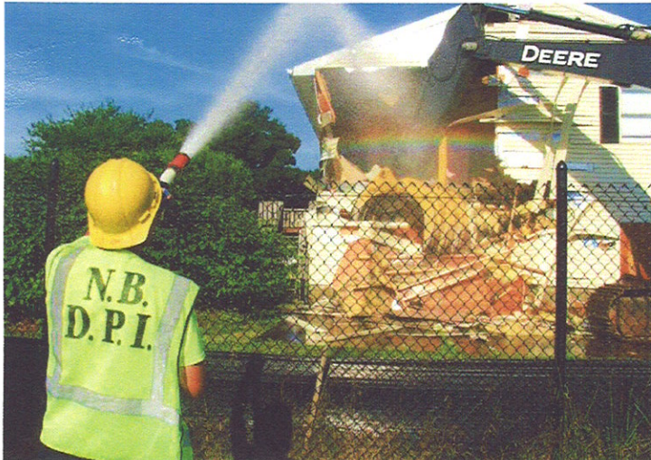
5. Active dust suppression during demolition (7/19/10).
