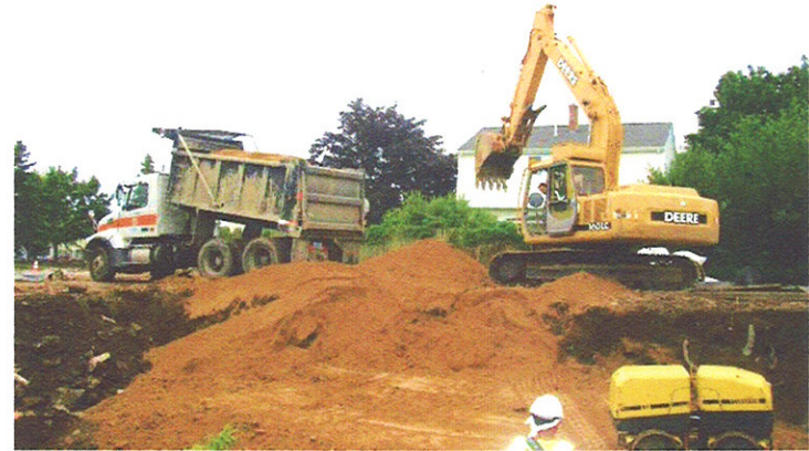
14. Backfilling and compacting at 118 Ruggles Street (7/23/10).
