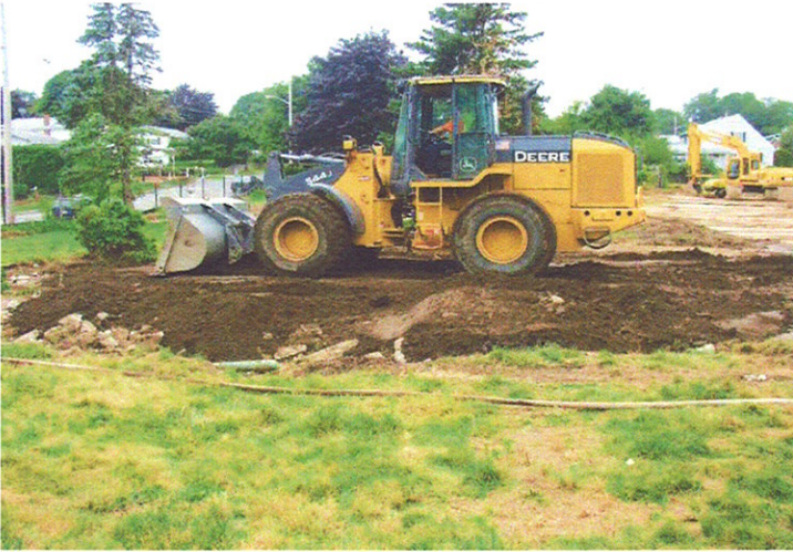
17. Spreading documented clean loam over top of backfilled foundation footprints (7/29/10).
