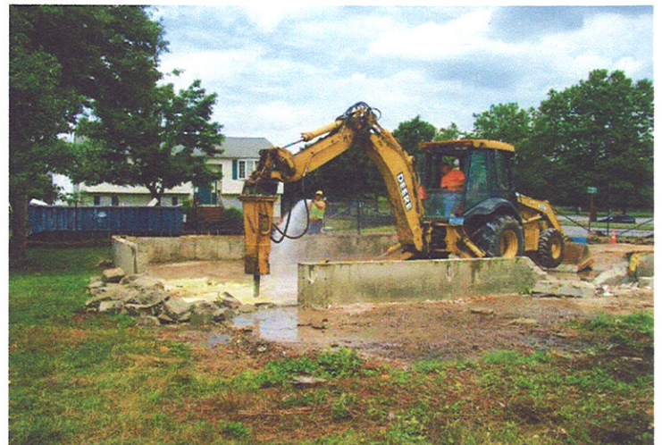
8. Hoe Ram breaking concrete at 102 Greenwood Street with active dust suppression (7/20/10).
