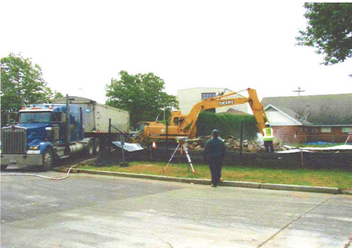
11. Loading concrete into trucks for offsite disposal (7/21/10).
