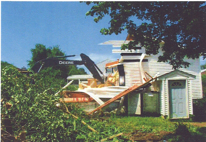
7. Beginning of structural demolition at 118 Ruggles Street (7/20/10).
