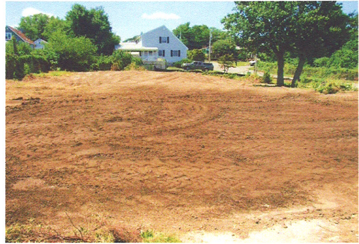
18. Finished grading in area of 108 & 118 Ruggles Street parcels (7/30/10).
