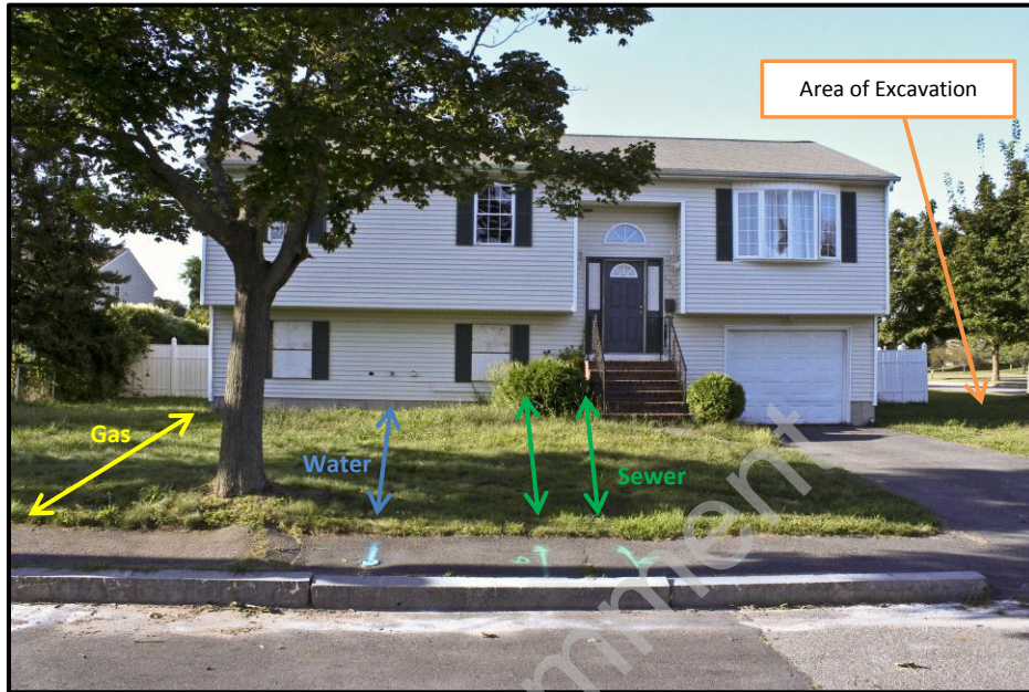
Photo 1 – Subsurface utility locations on south side of property (101 Greenwood Street)
