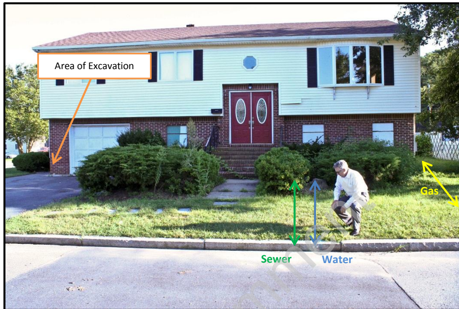
Photo 3 – Subsurface utility locations (102 Greenwood Street)
