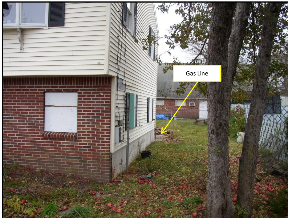
Photo 4 – Location of gas line on west side of property (102 Greenwood Street)
