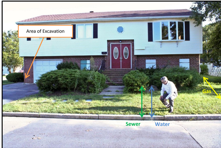
Photo 3 – Subsurface utility locations (102 Greenwood Street)
