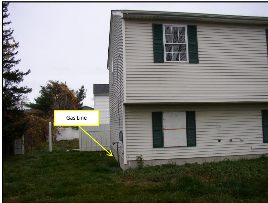
Photo 2 – Location of gas line on west side of property (101 Greenwood Street)
