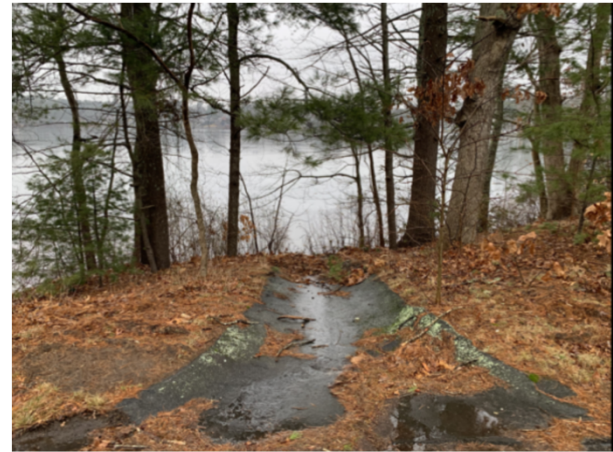
SW-1 (Sassaquin Ave. at Thrush St.)
