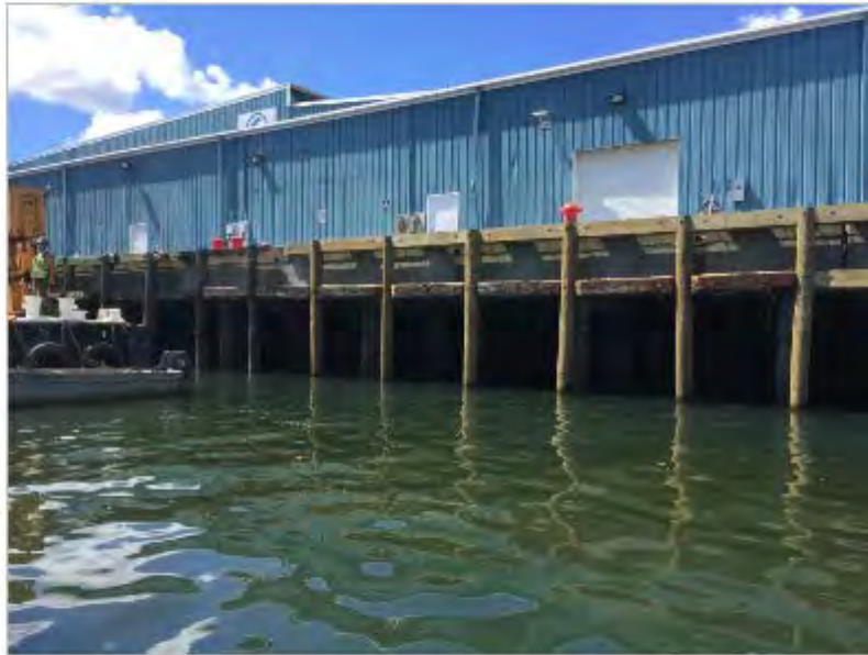
Photograph 4: Replaced timber fender along Seawatch parcel
