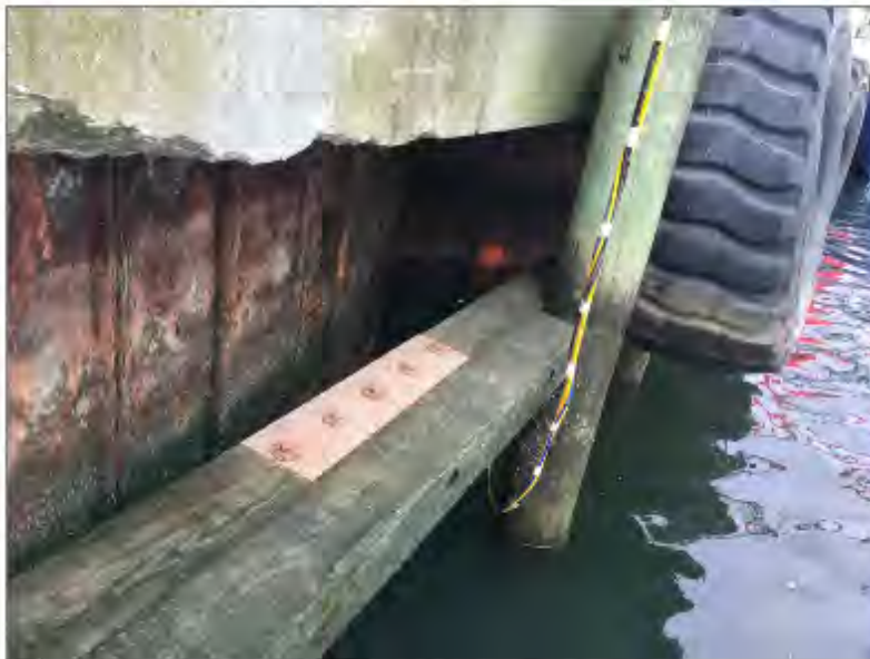
Photograph 3: Typical bulkhead/fender construction
