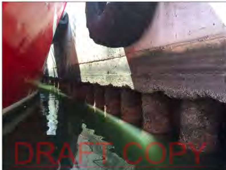
Photograph 1: Typical pile layout along fender line
