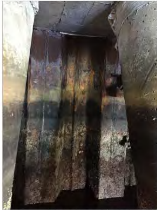
Photograph 11: Typical Sheet Pile Condition
