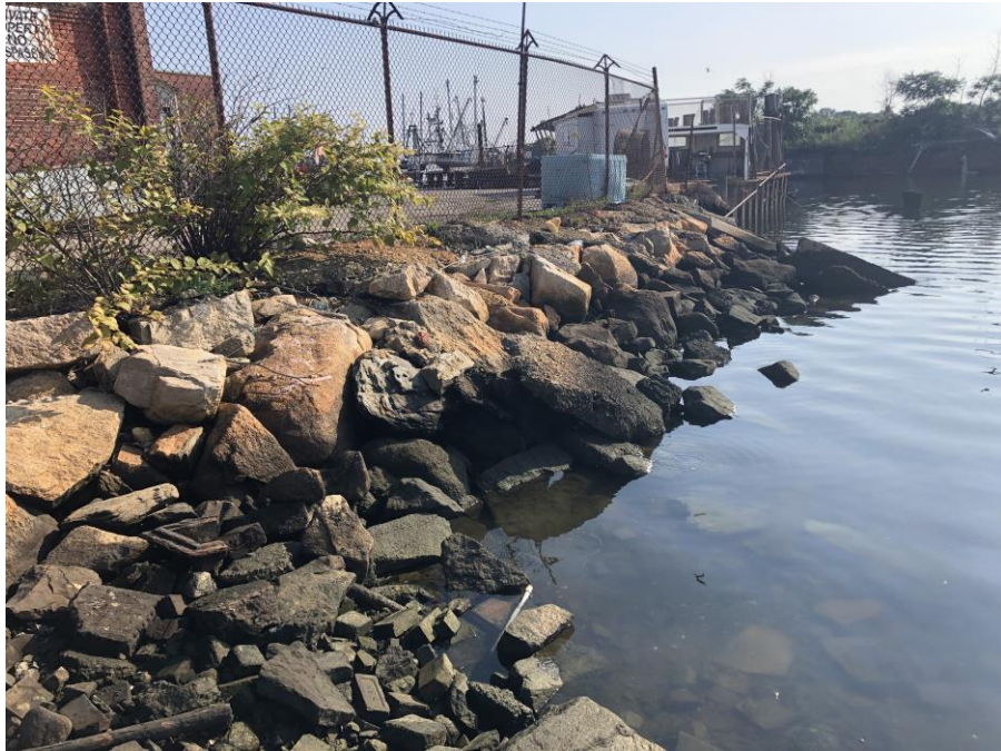
Photo 4 – South Timber Bulkhead/Revetment
