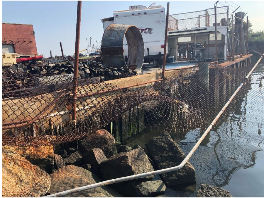
Photo 3 – South Steel Sheet Pile Bulkhead
