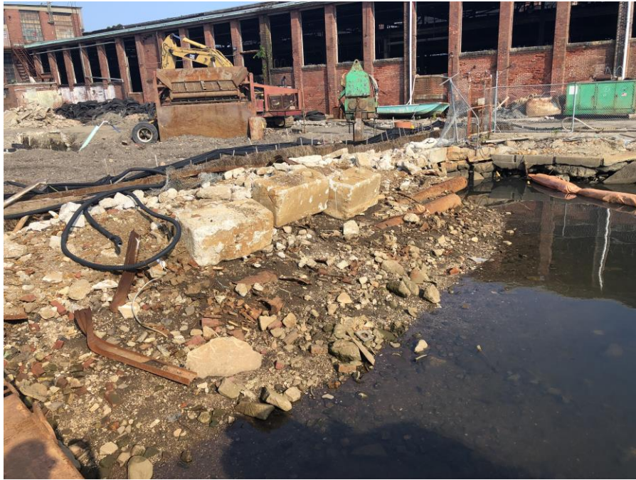
Photo 1 – South Revetment Area
