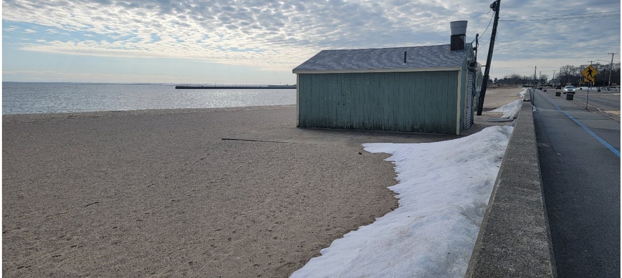
Photo 9: South view of East Beach from sea wall with northern wooden structure.
