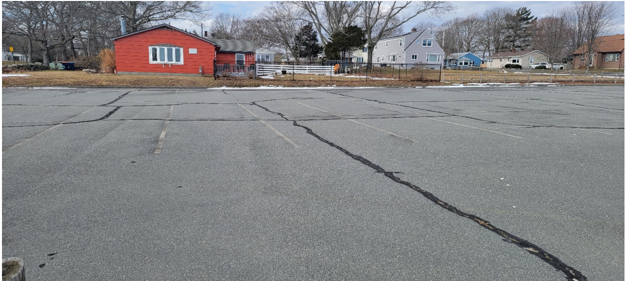
Photo 1: Southwest view of southernmost parking lot from East Rodney French Boulevard.
