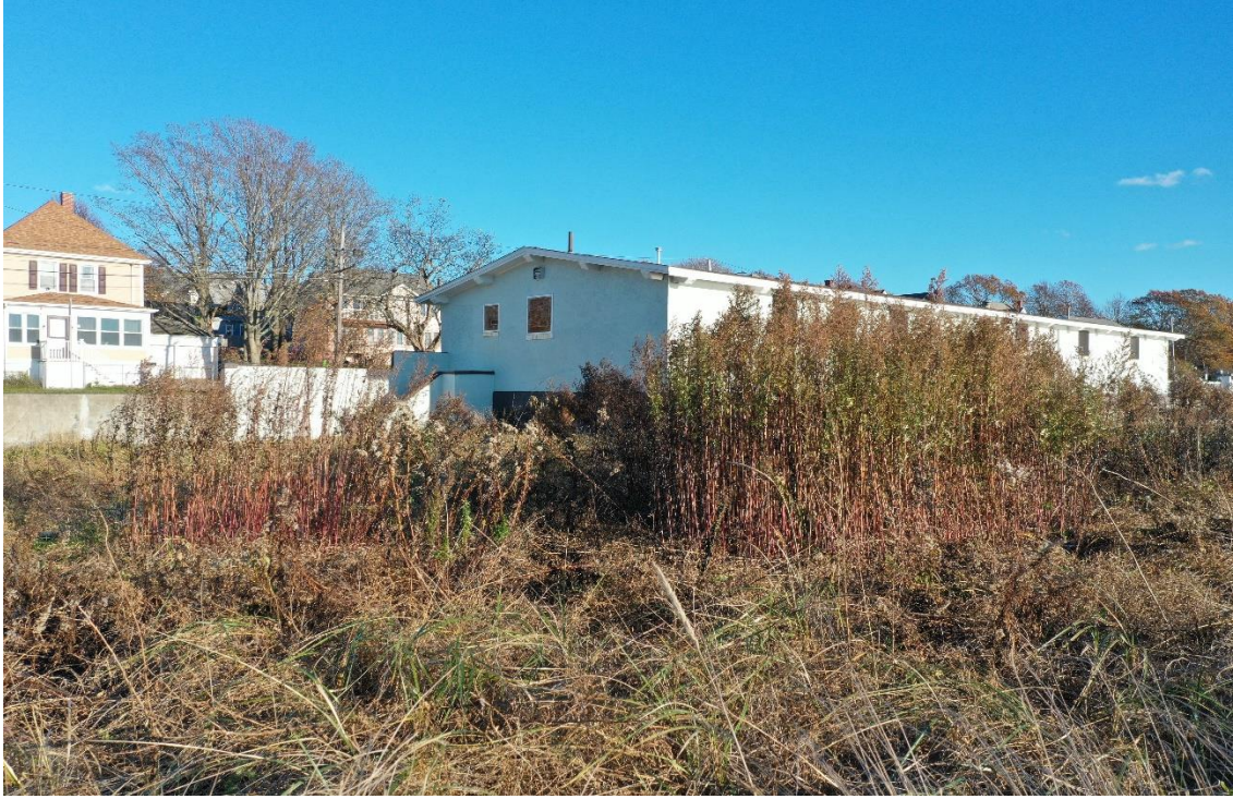
Photo 3: Field view of area 1. Fall 2021
