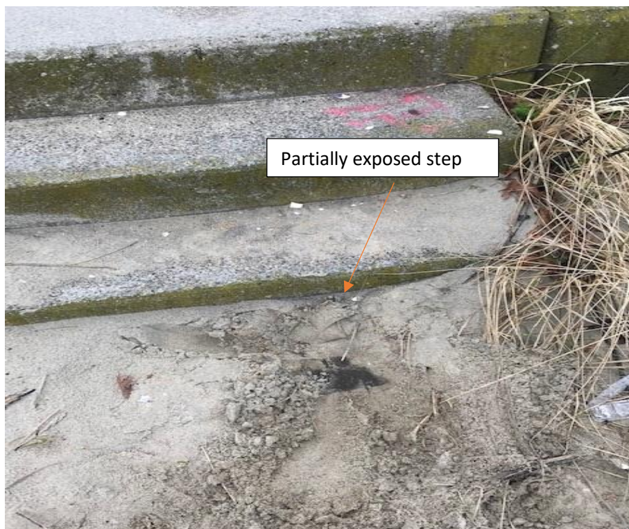
Photo 5: Close up of the existing steps at Squid Beach
