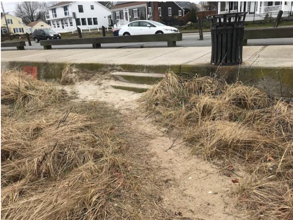
Photo 4: Squid Beach steps. Minor grading (hand shovel) will take place to expose the existing steps.
