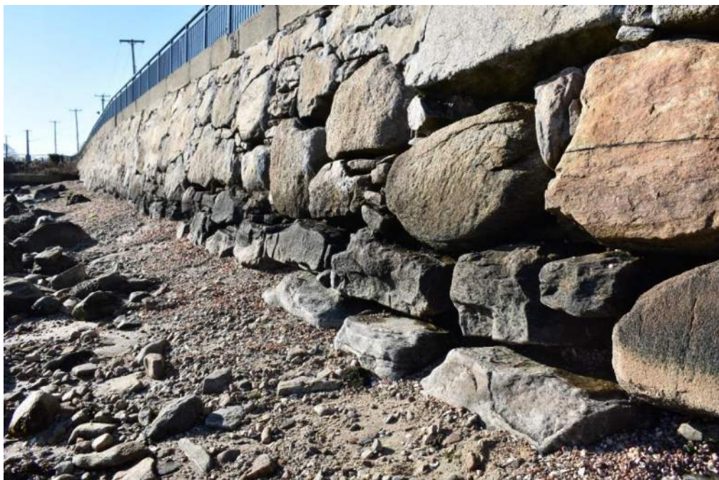
Photo 13: Face of wall looking south
