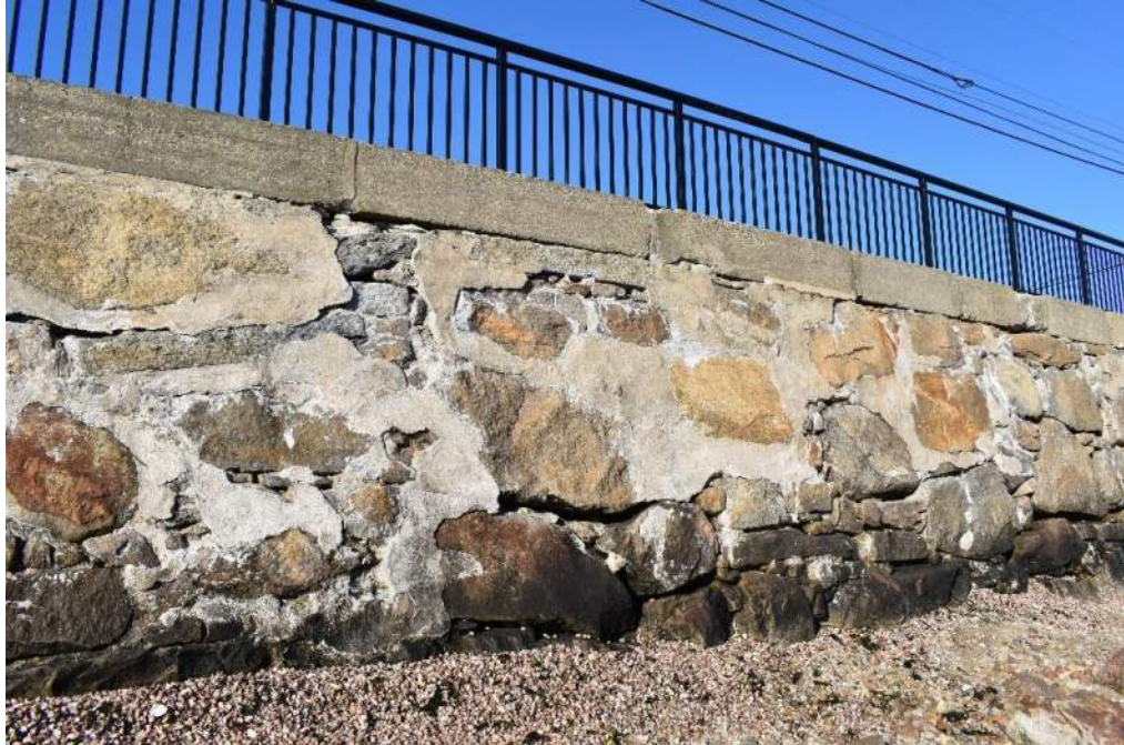
Photo 11: Face of wall
