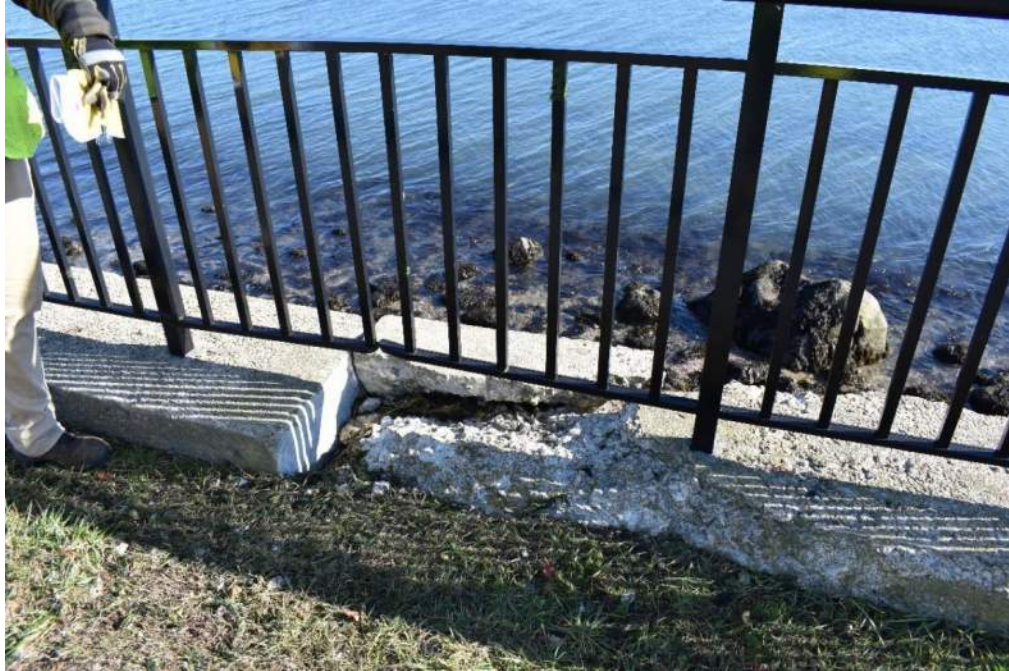
Photo 25: Concrete cap and fence
