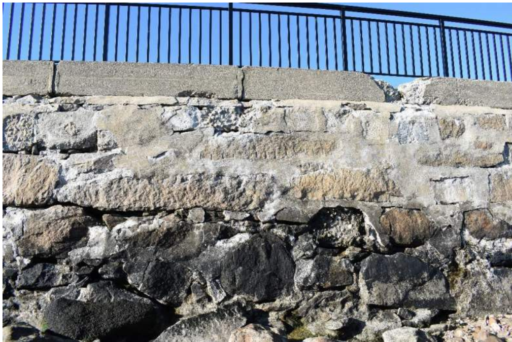
Photo 16: Face of wall
