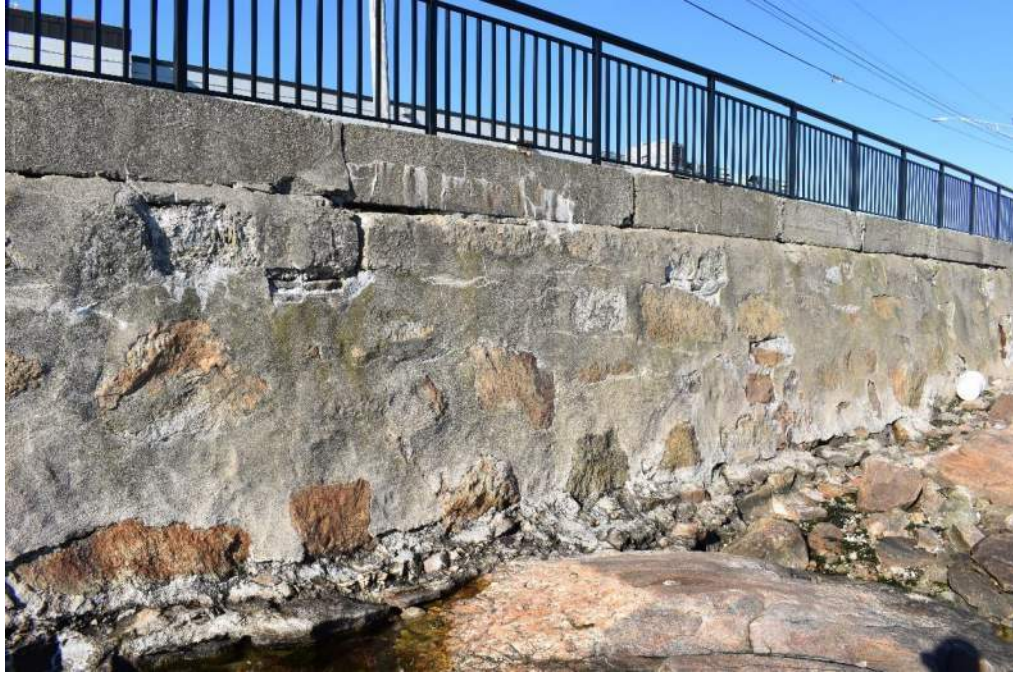
Photo 17: Face of wall
