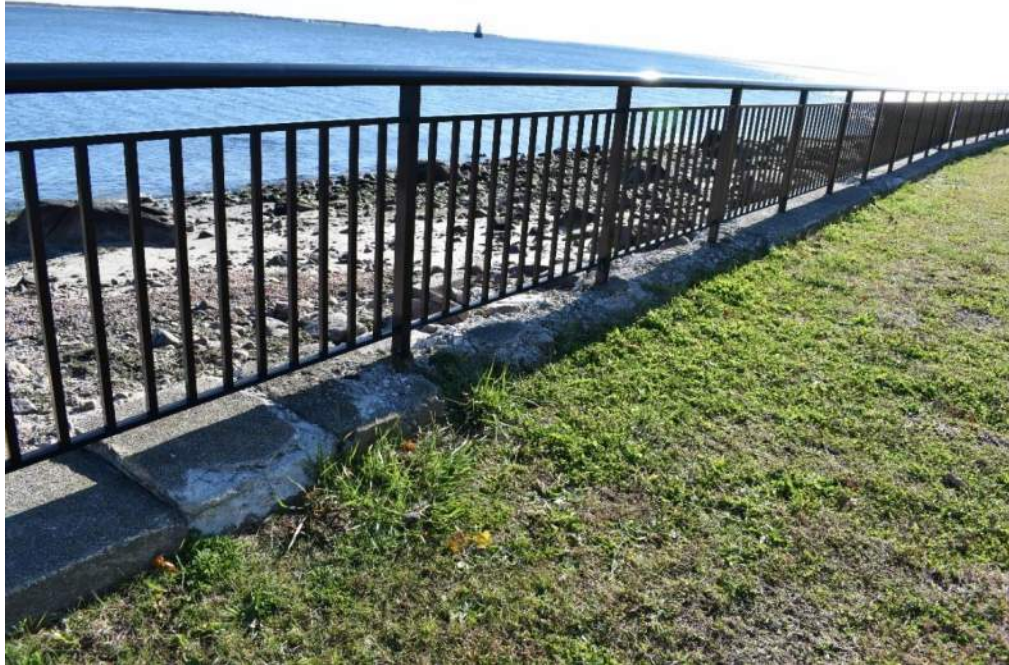
Photo 23: Concrete cap and fence
