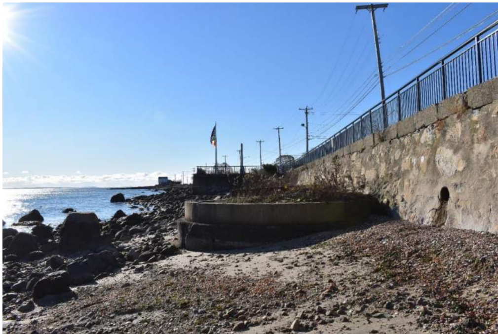
Photo 10: Face of wall looking south
