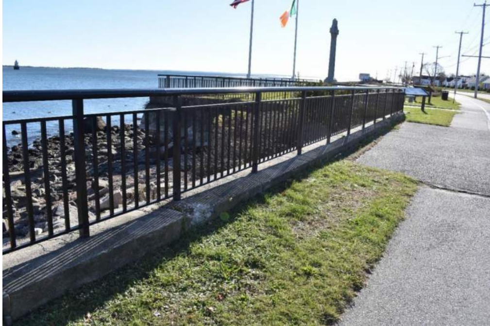
Photo 27: Concrete cap and fence
