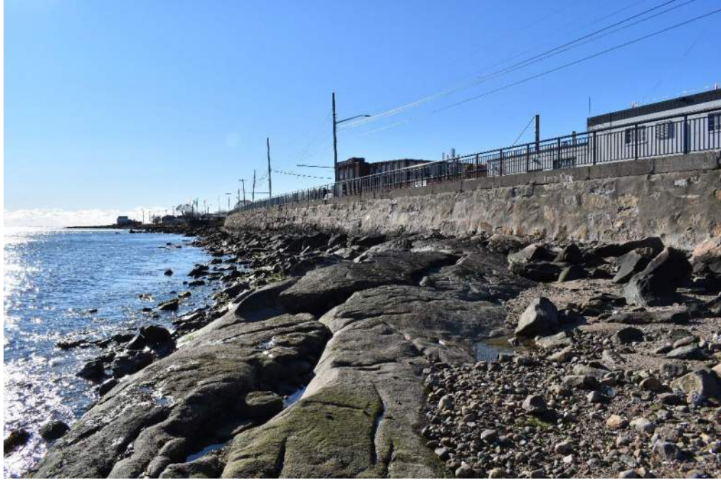
Photo 19: Face of wall looking south
