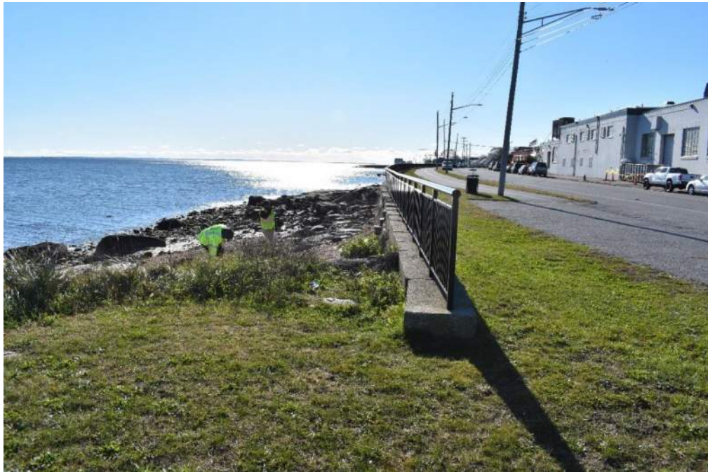
Photo 22: Concrete cap and fence
