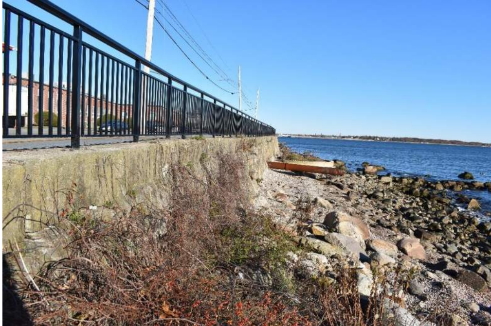
Photo 7: Face of wall looking North
