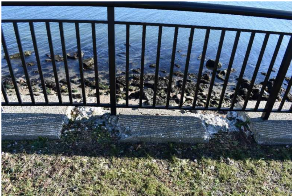
Photo 24: Concrete cap and fence
