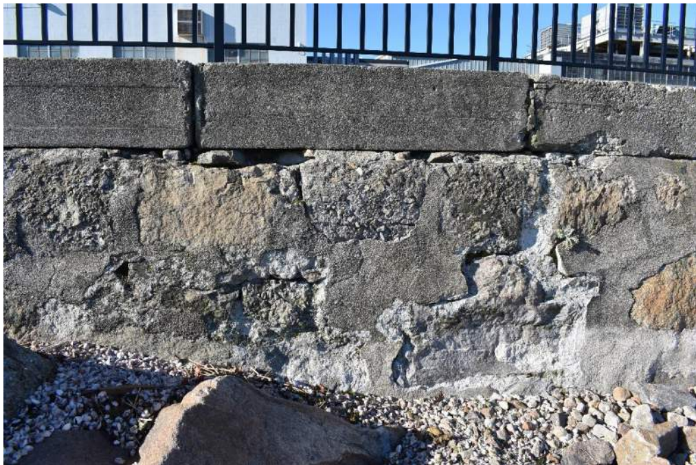
Photo 20: Face of wall and concrete cap
