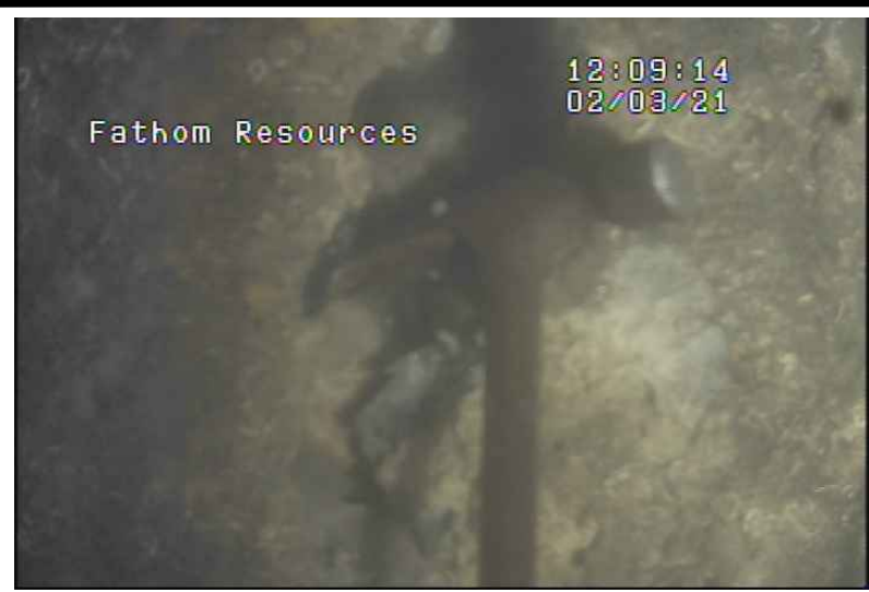
CELL #1: HOLE 4' X 6' @ TOP NEAR CONC. CAP INTERFACE
