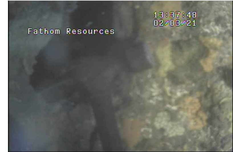
CELL #5: HOLE 2' X 2' @ TOP BY DIVER
