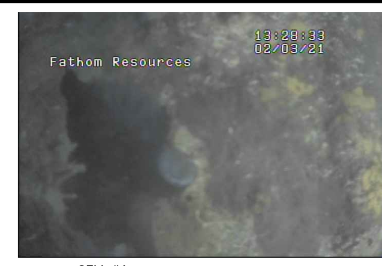
CELL #4: HOLE 6' X 10' @ TOP @ EXPANSION JOINT
