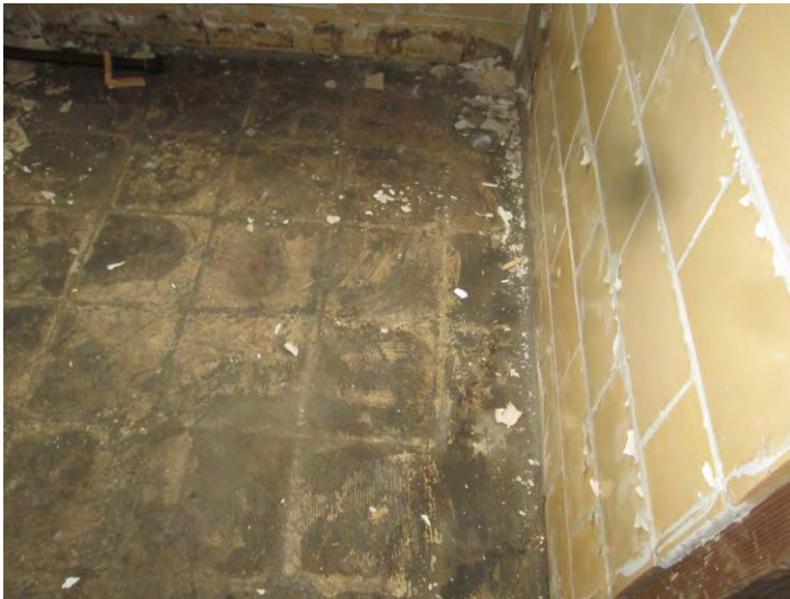
Photo 2 Typical view of the black mastic located in the 1st floor locker room and adjoining rooms of Building 1.
