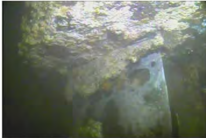
Photograph 7: Bent 16 Pile C2 - Bottom of concrete jacket visible
