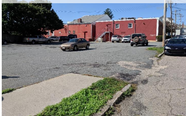
Parking lot & driveway (looking west from Taber St)
