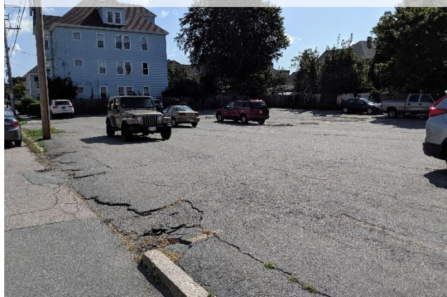
Parking lot & driveway (looking east from Taber St)
