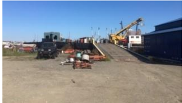
Ramp Providing Access to the Docked Barge
