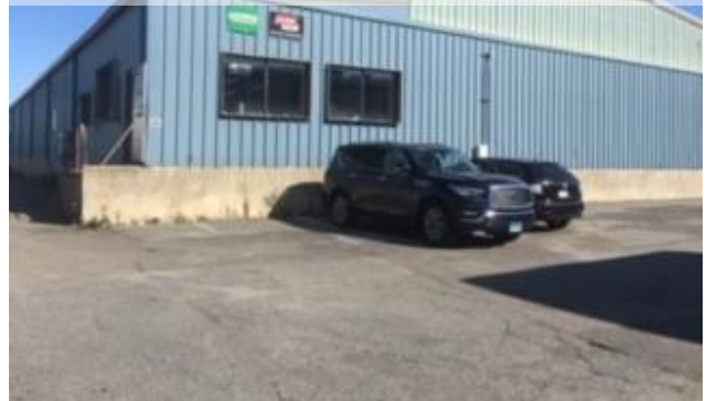
143 Popes Island – East Coast Fabrication Building
