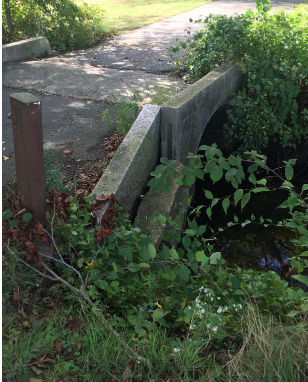
Concrete Bridge - Northwest Area of North Woods
