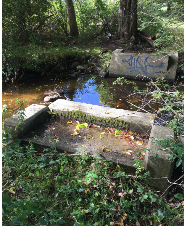
Concrete Bridge - Southwest Area of North Woods
