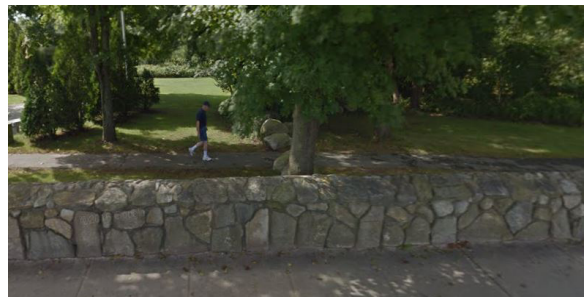
Stone Wall Along Route 6
