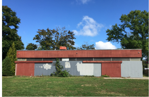
Joseph F. Waldron Barracks Veteran's Memorial Building
