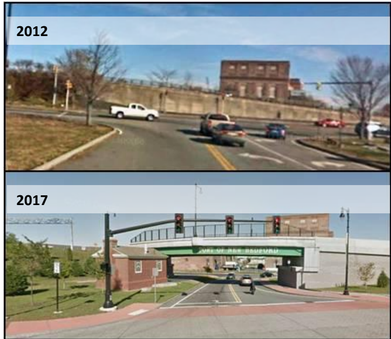
Northeast Corner of Elm St and Route 18: Before & After Roadway Reconstruction
