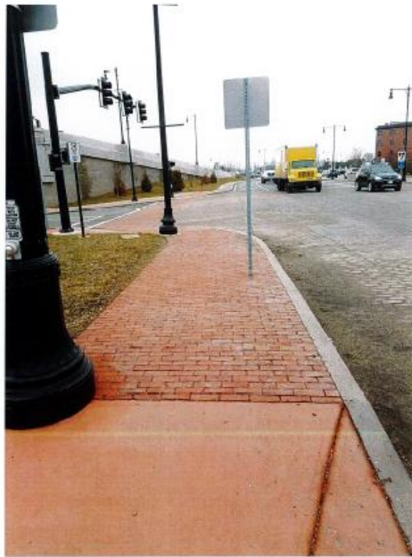
STAINED CONCRETE AND BRICK SIDEWALKS
