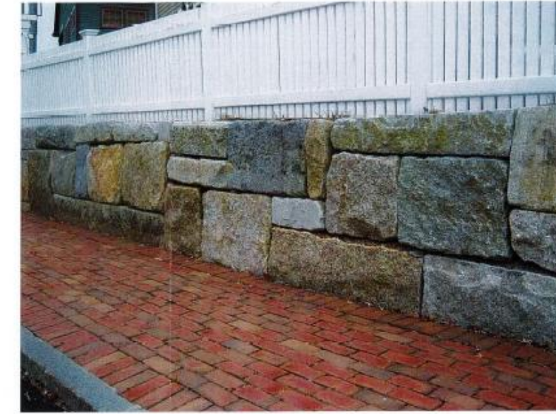
GRANITE BLOCK RETAINING WALL
