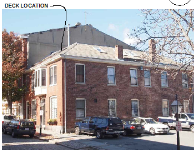
VIEW FROM HAMILTON STREET
