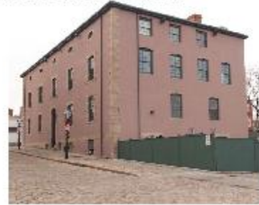
72 N. Water St., East (Rt. 18) Elevation.
