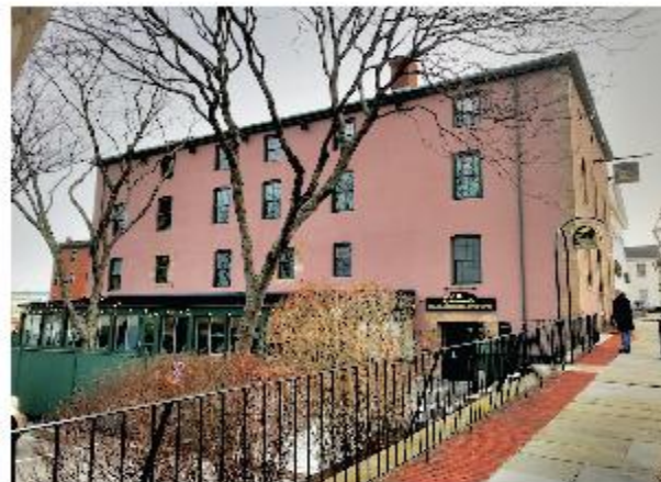
Candleworks Building, as seen from Water Street.
