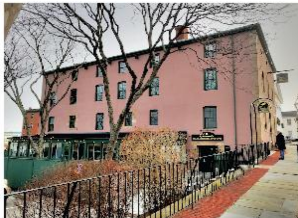
Candleworks Building, as seen from Water Street.
