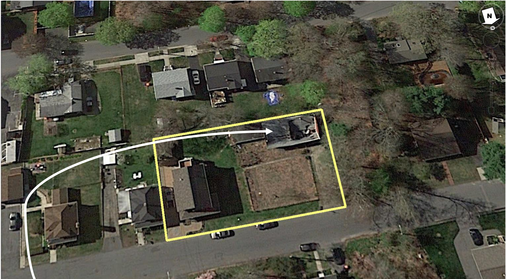
1024 Sheffield Street (Map: 132H, Lot: 182) collapsed roof shown Google earth
