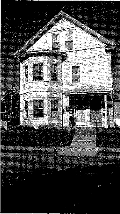
33 Front of Building
