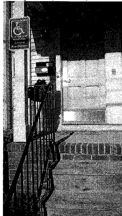
28 Front Entry: 8' From Sidewalk
