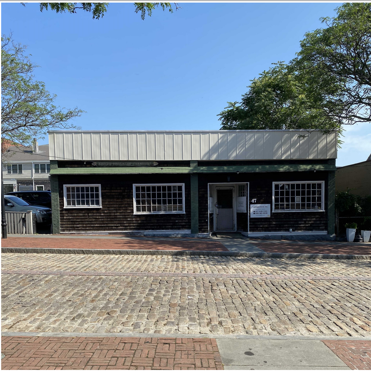
FRONT VIEW EXISTING
