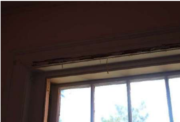
1. Interior - Moisture damaged plaster at window head.
