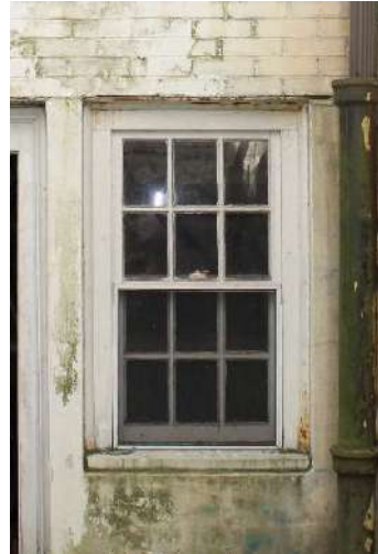
4. Exterior light well – rusty steel lintel, algae and weak masonry joints at window.
