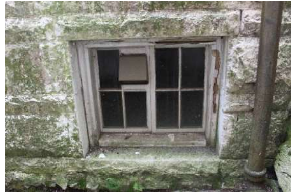
6. Basement – Damaged window frame and sash conditions.
