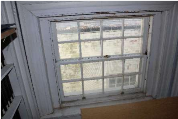
5. Law library – Moisture damage at window casing & sash.
