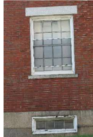
12. Typical conditions of windows in masonry wall.
