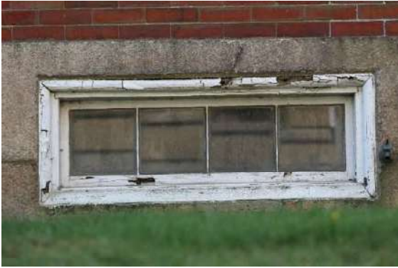
3. Exterior – deteriorated wood window casing at basement level.
