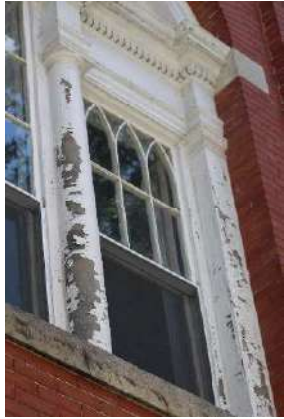
9. Westside moisture damage to paint @ ceremonial stair window.
