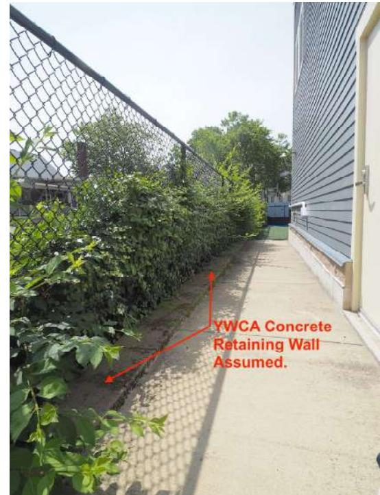
Additionally, the Nativity Prep side of the eastern retaining wall appears to be a stone wall facing east. We see evidence of granite stones, and the excessive growth abruptly stops at the termination of the concrete retaining wall of Nativity Prep play area. We assume that the growth is occurring in the crevasses of the stone wall, and potentially causing damage to the structure. We recommend removing the growth, examining the stone wall, and repairing/repointing the masonry.
