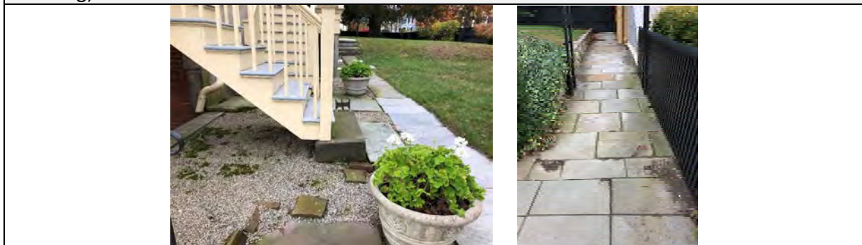
Fig. 38 North elevation showing displaced granite steps (shedding water south toward building)
