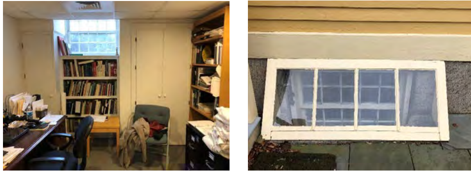
Fig. 36 Windows: North room, cellar window/well that is not weathertight and allowing water into the building's basement (center) office, near electrical panels
