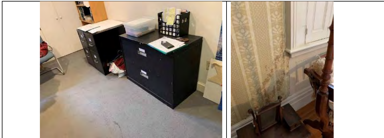
Fig. 20 Prior leaks into the curators office have fostered an embedded mold colonization in the rug (left). Building breaches have also contributed to water seepage creating stains on wallpaper (right).
