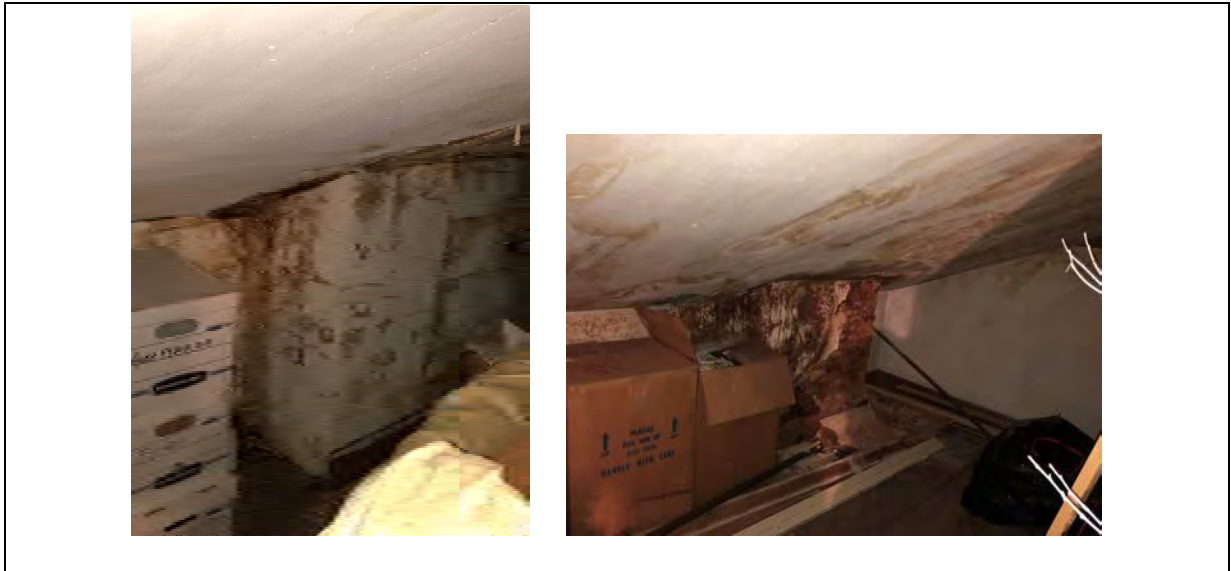
Fig. 29 Chimney: Typical conditions of chimneys in attic, including damage from water intrusion around the chimney, resulting in creosote-staining as well as failing plaster parging.
