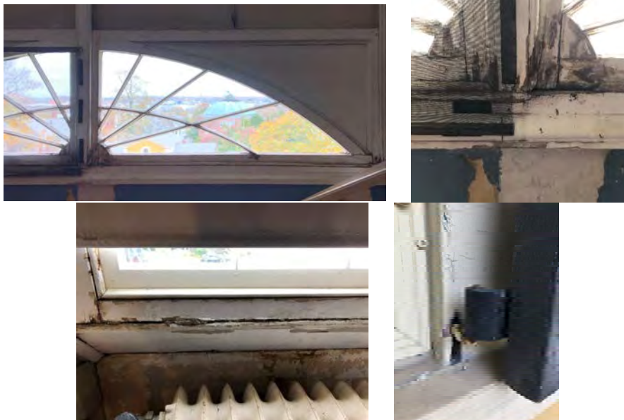
Fig. 37 Windows: Typical window conditions that need repair
