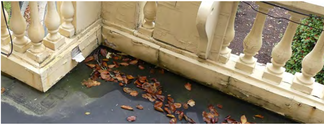
Fig. 34 Woodwork: West façade balustrade needing repair and re-painting
