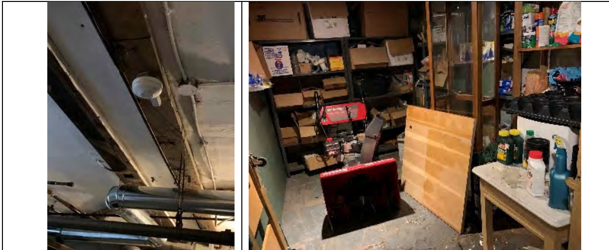
Fig. 21 Hard wired smoke detectors are in place. A basement mixed facility space adjacent to the furnace room presents a fire hazard.
