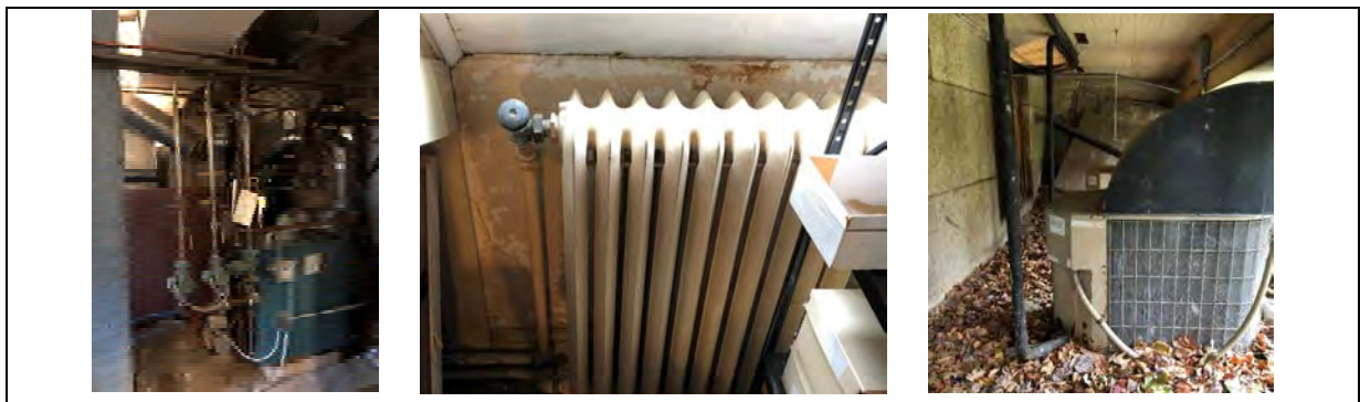
Fig. 40 HVAC: Furnaces in basement, steam radiator in attic, and AC condensers under north porch
