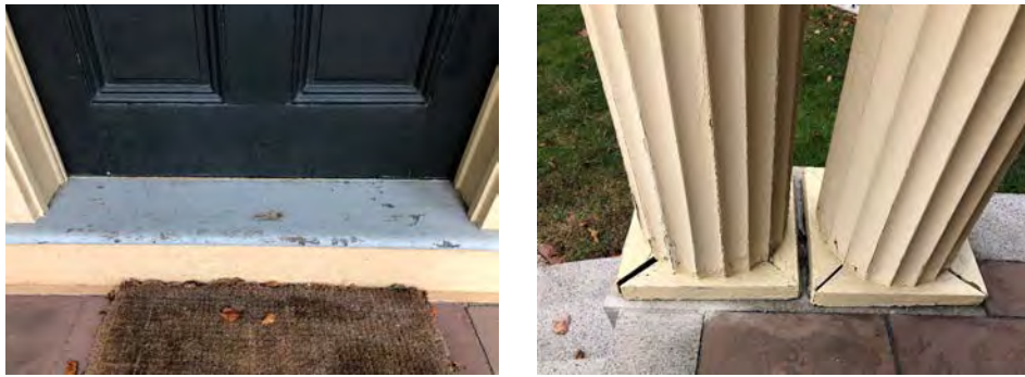
Fig. 33 Woodwork: Conditions needing repair/re-painting
