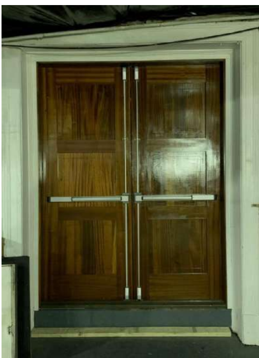
Interior north elevation new emergency egress doors, facing N.
