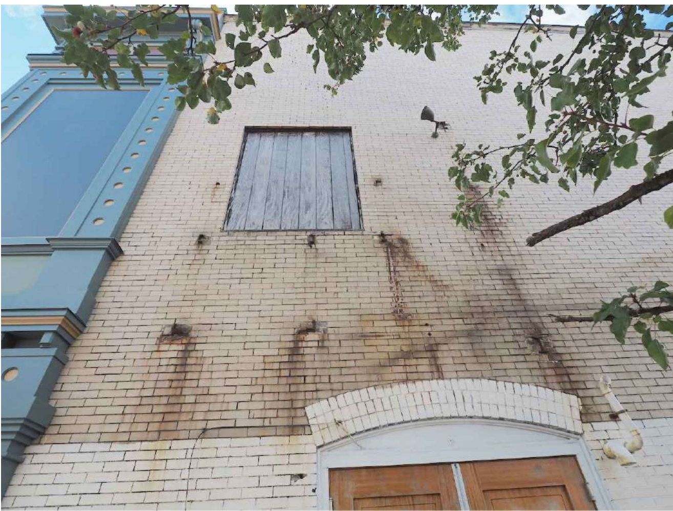
PHOTO 2: NOTE 4 REPAIR AT FASTENERS SCALE: N.T.S.
