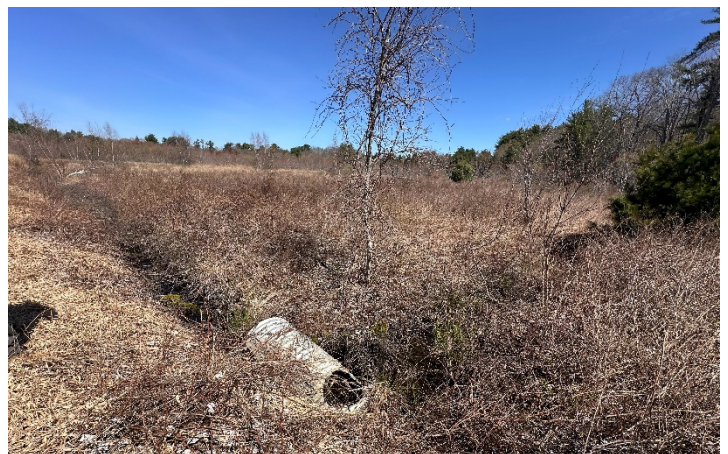
Damaged and abandoned infrastructure in the bogs. Looking west from the east side of the site.
