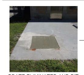
**GRATE ELIMINATED AND PIT** FILLED AND CAPPED IN **CONJUNCTION WITH** VENTING **RE-CONFIGURATION**
