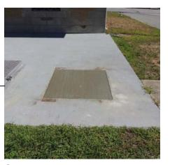
**GRATE ELIMINATED AND PIT** FILLED AND CAPPED IN **CONJUNCTION WITH** VENTING **RE-CONFIGURATION**
